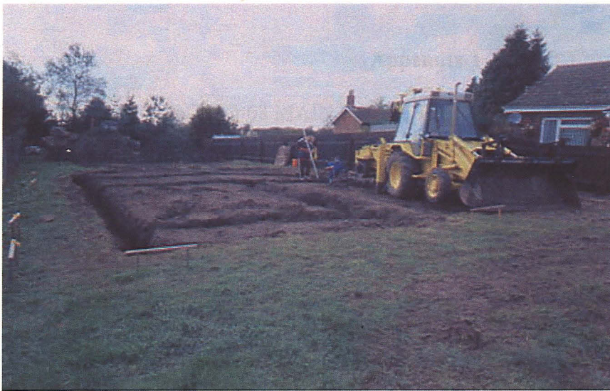
Plate 1 - General view across the development area, looking northwest
