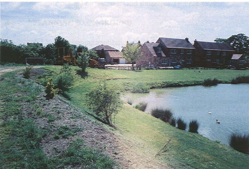
Plate 8 - View showing the completed plots 1 and 2, looking southwest
