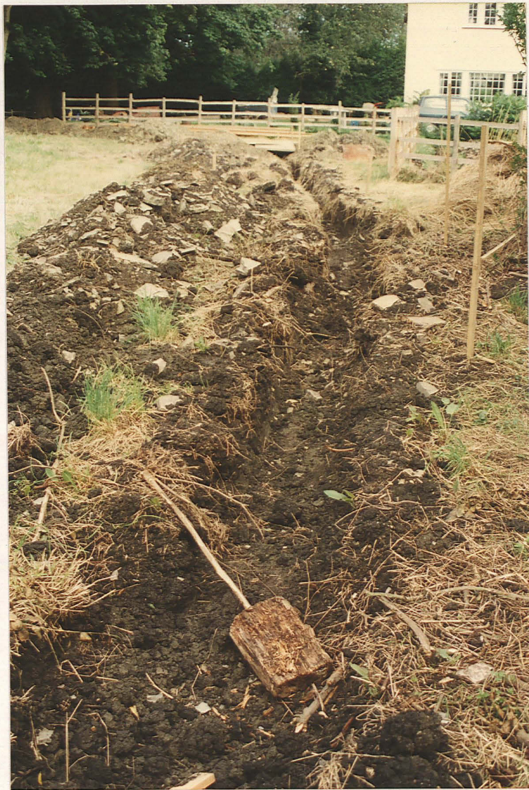
Pl. 3 Sewage pipe trench along east boundary of site, looking north.
