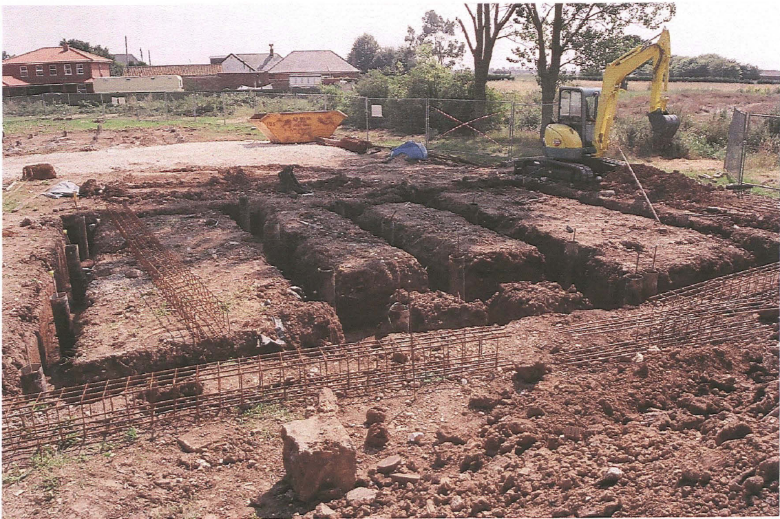
Pl. 2 View of house foundations A/B looking south
