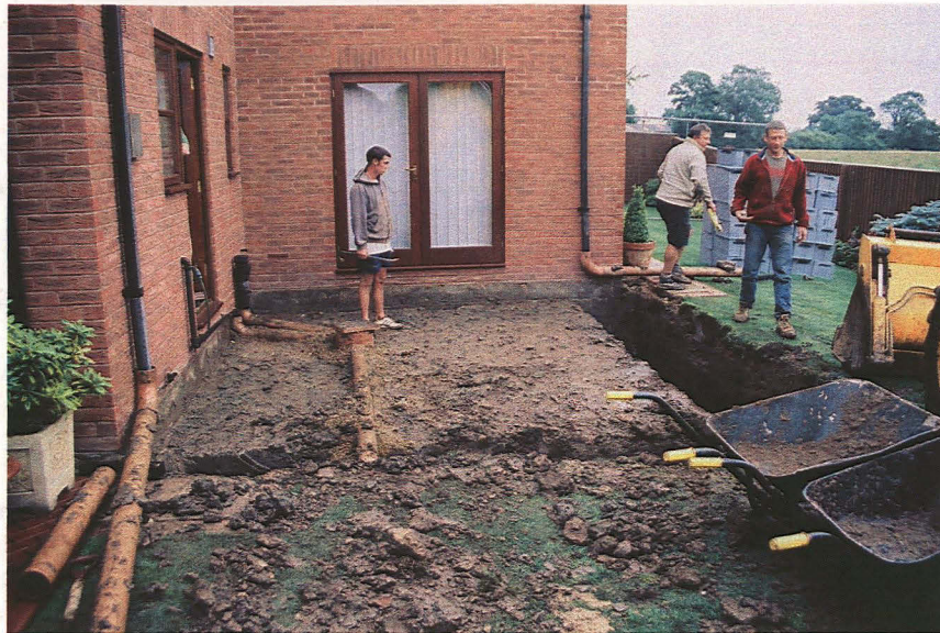
Plate 1 - View showing the completed foundation trenches, looking northeast
