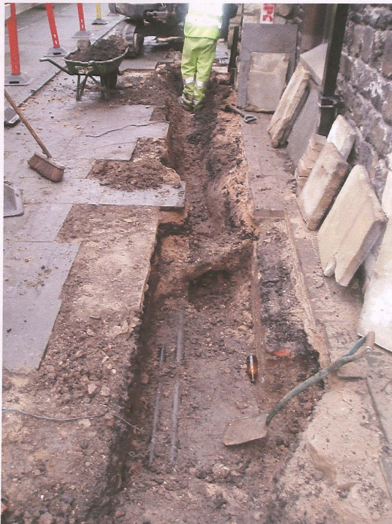
Pl. 10 Observation Point 15 showing existing pipes at base of trench.
