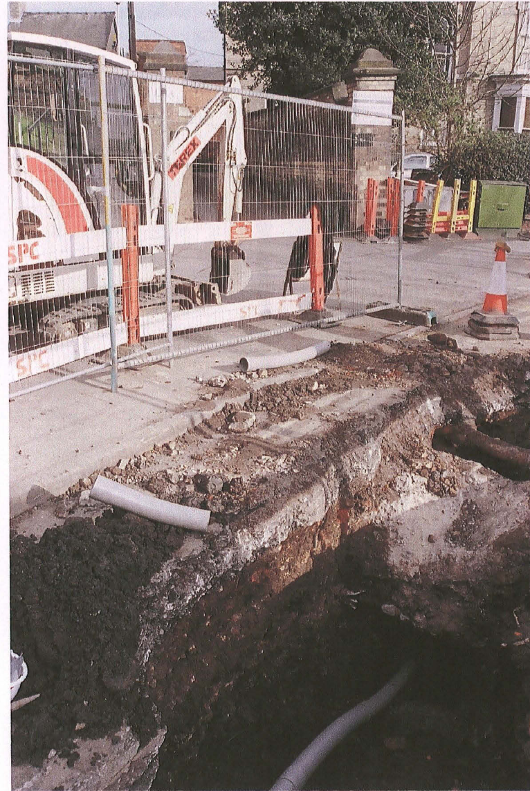
PI. 4 Observation Point 8 deposits at Newland outside No. 29.
