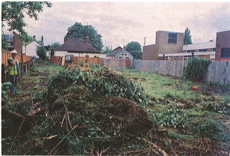
Plate 2 General view of the site, looking southwest
