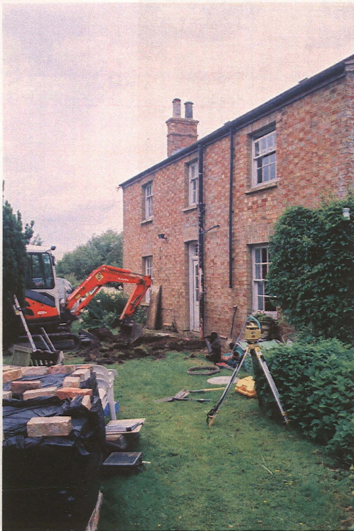
Plate 2 General view, excavation in progress.
