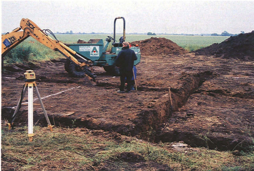
Plate 1 - View across the site showing the foundation trenches, looking northwest
