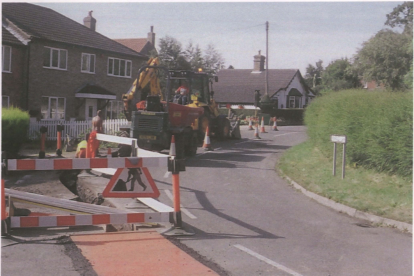
Pl. 6 Work progressing along Pinfold Lane
