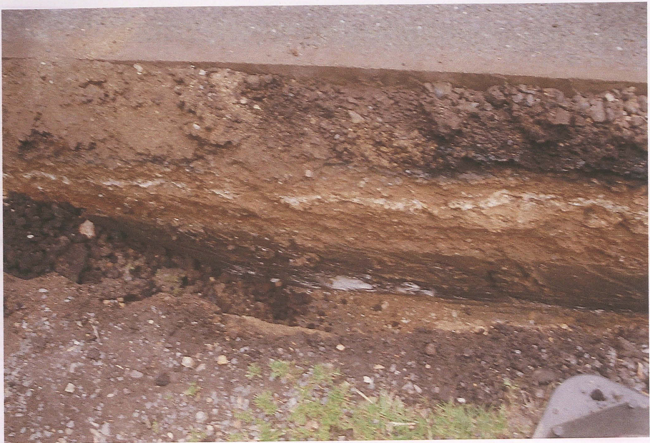
Pl. 3 Trenching along Pinfold Lane
