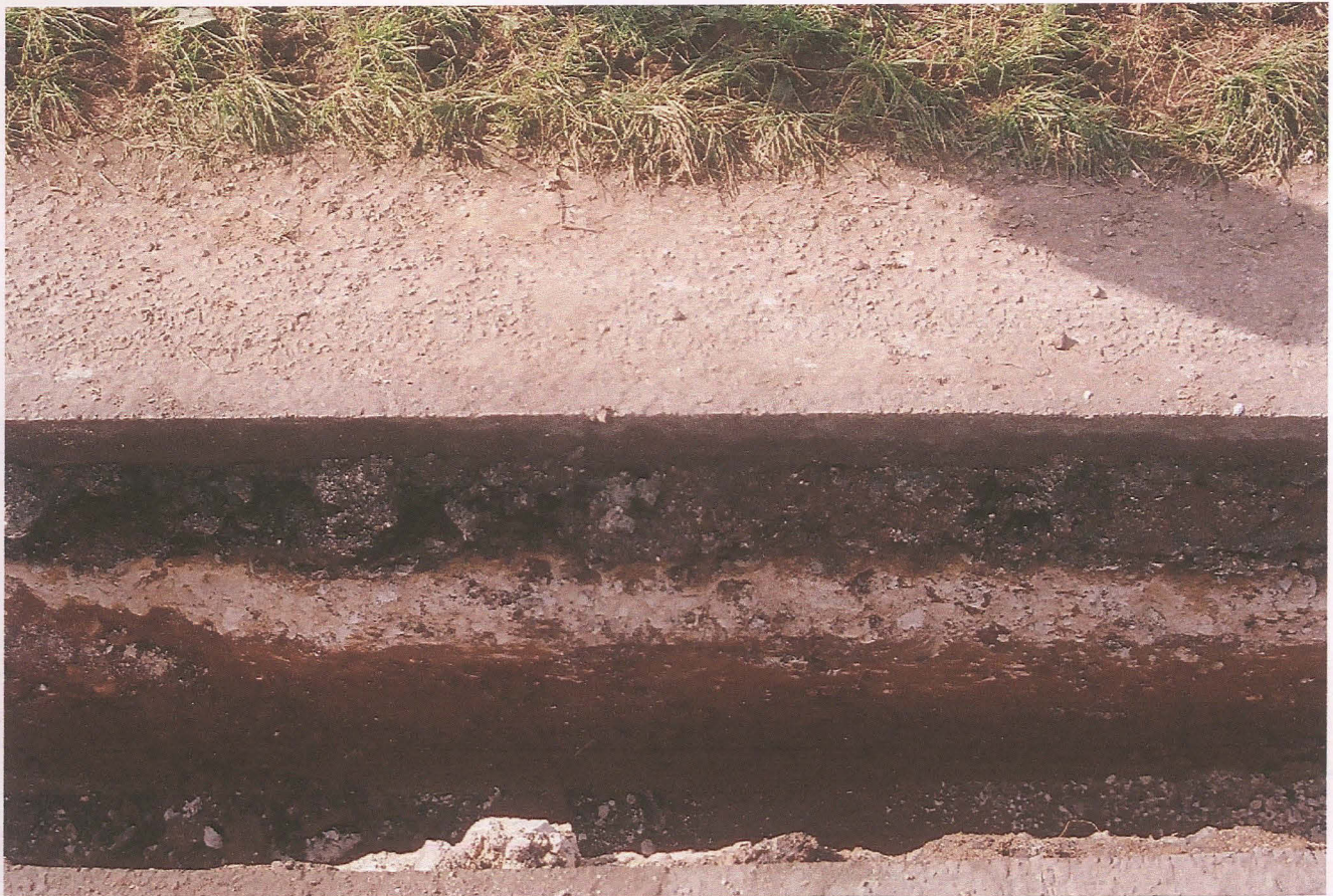
Pl. 8 Road build-up sealing red brown clay along Top Road
