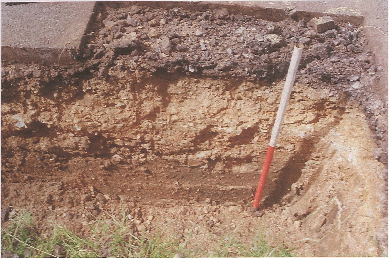
Pl. 5 Road build-up and clay subsoil on Pinfold Lane
