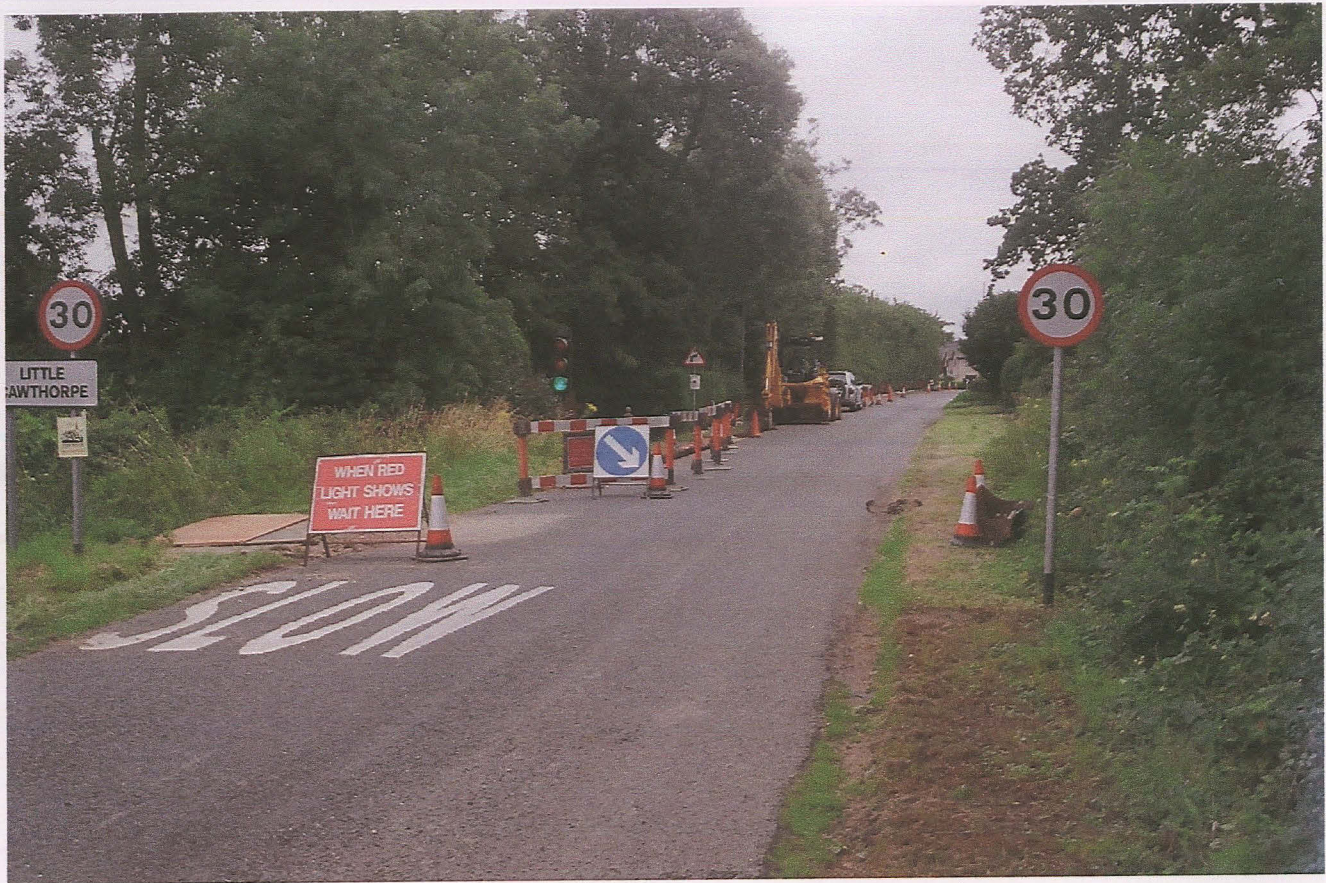
Pl. 1 Looking south along Planting Side prior to any works
