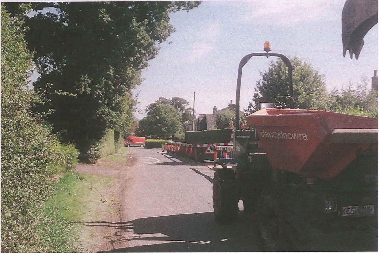
Pl. 7 Looking north along Pinfold Lane during excavations
