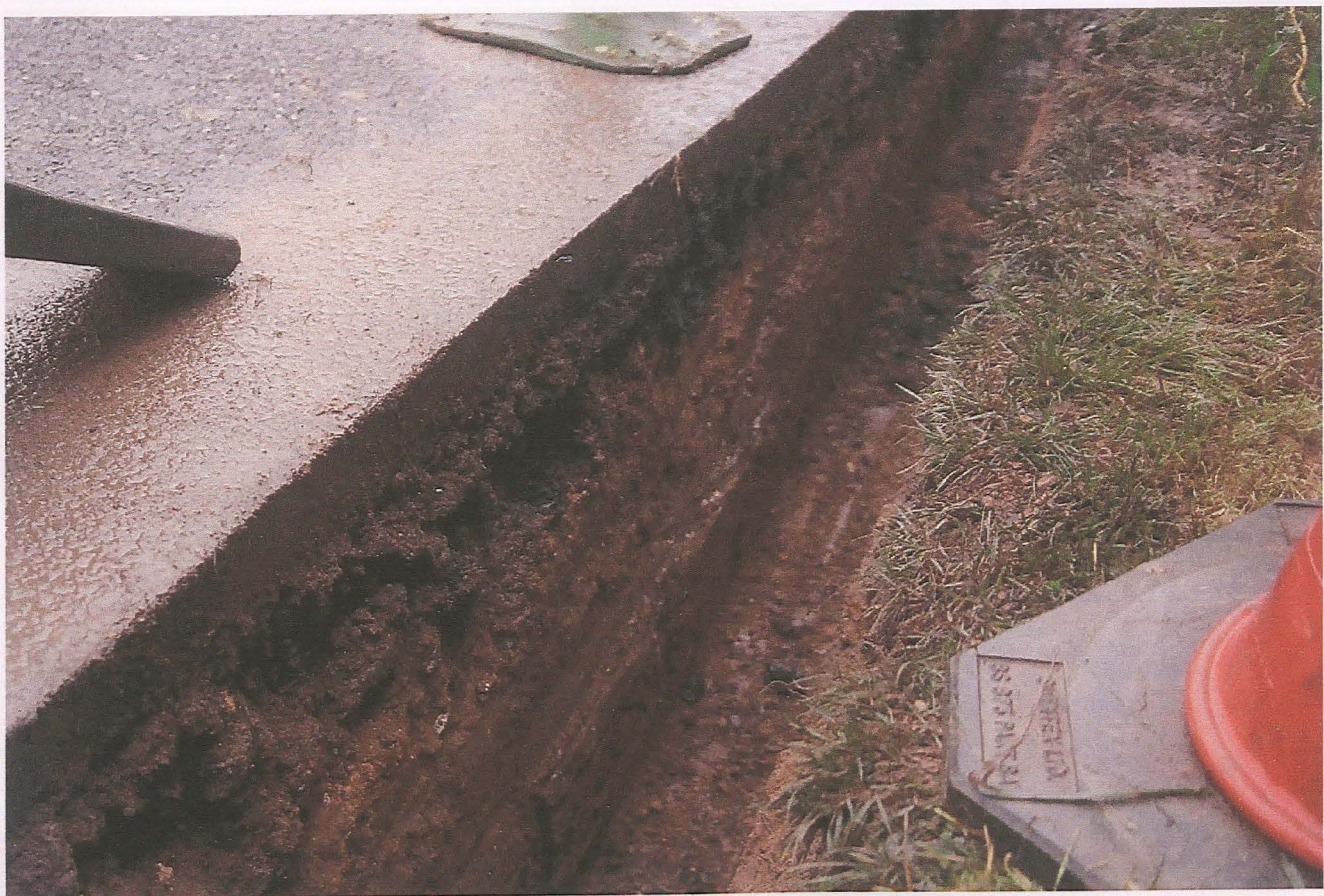
Pl. 2 Trenching along Planting Side
