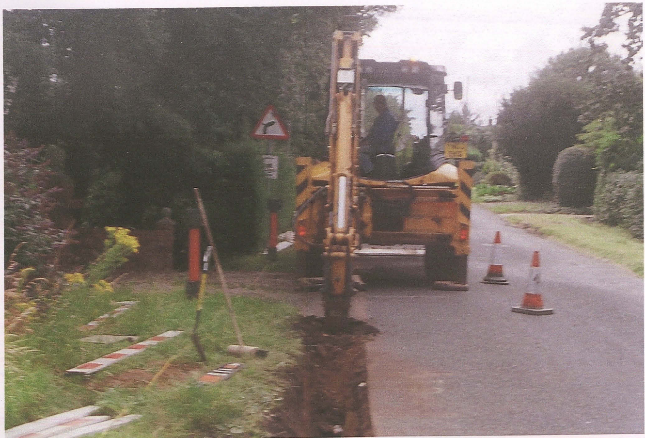
Pl. 4 Excavations along Planting Side
