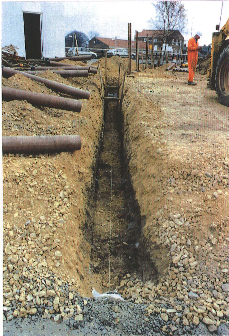
Photo. 3 Trench from interceptor tank to Horncastle Road, looking south-south-east
