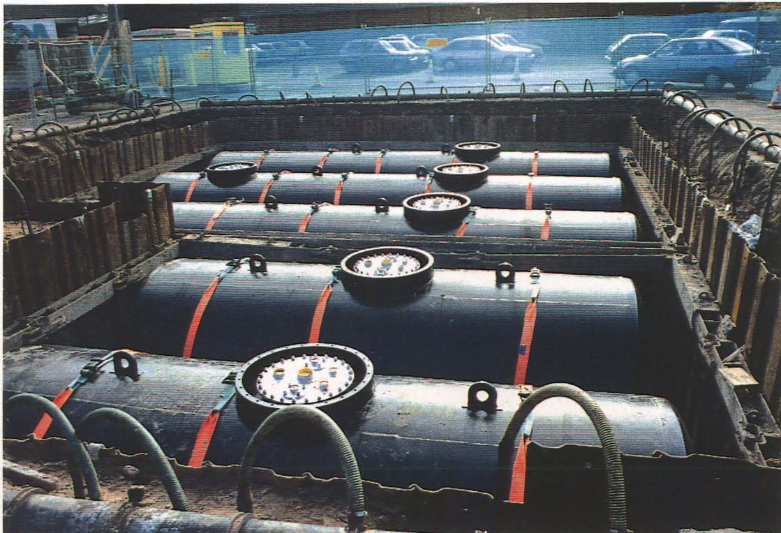
Photo. 2 Deep excavation cutting after shoring and insertion of new storage tanks.
