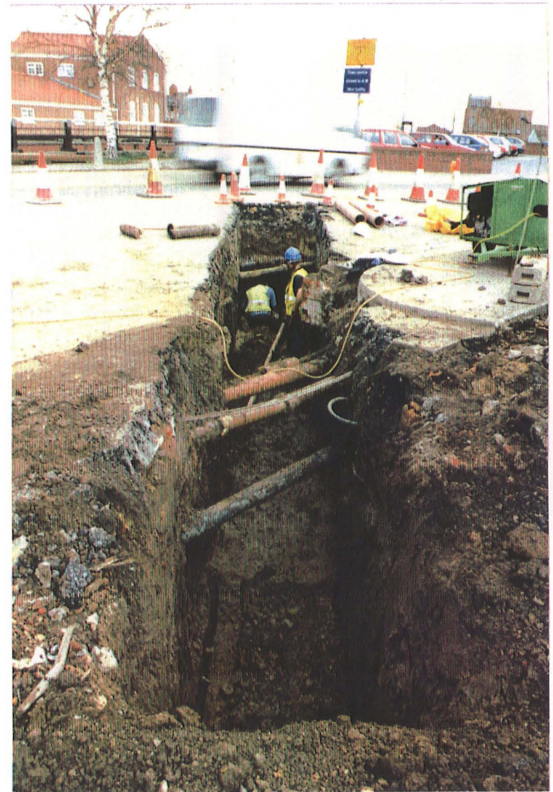
Photo. 4 Looking south into phase II road trench.
