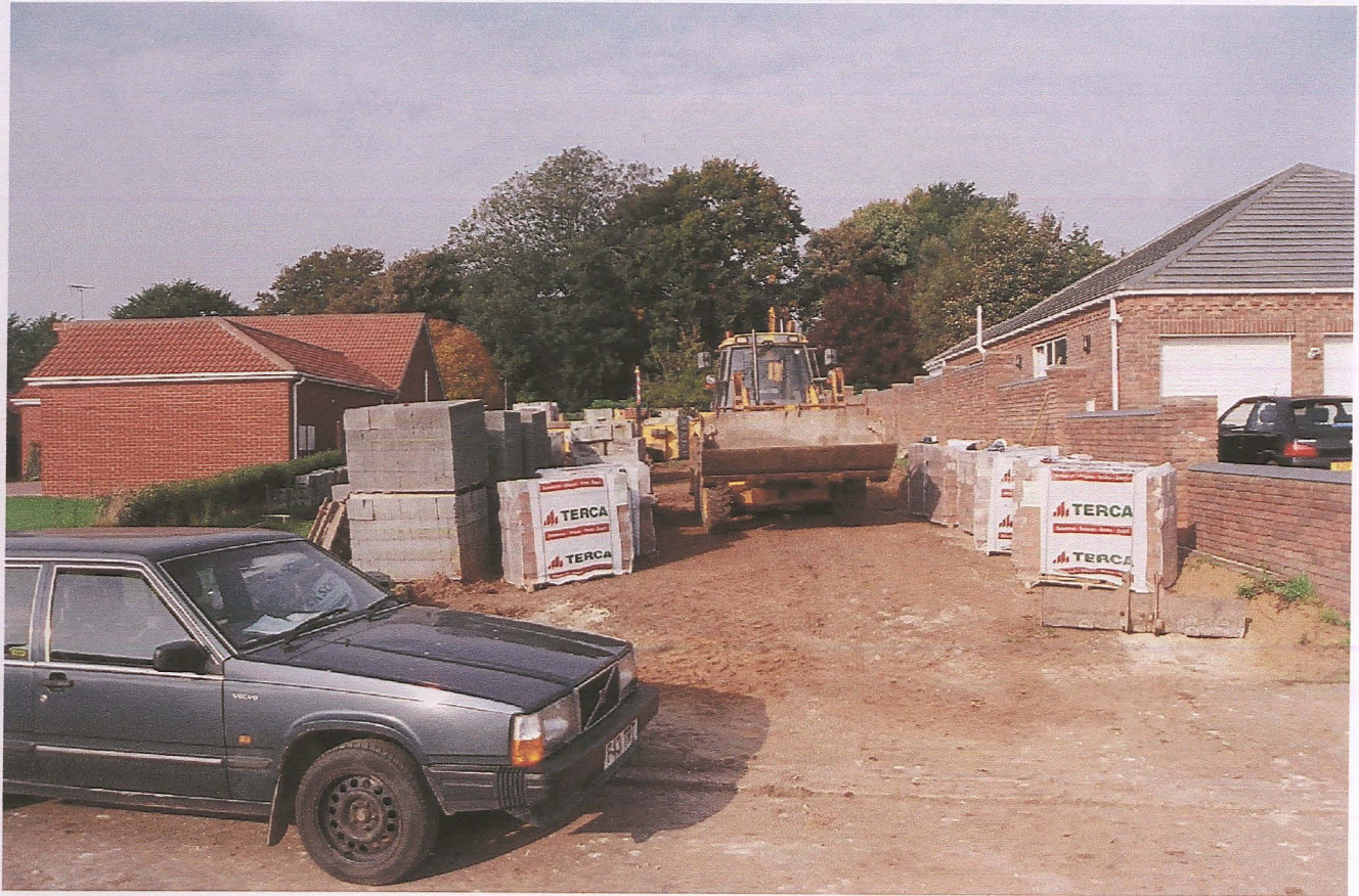
Pl. 1 Looking west across the site prior to any works
