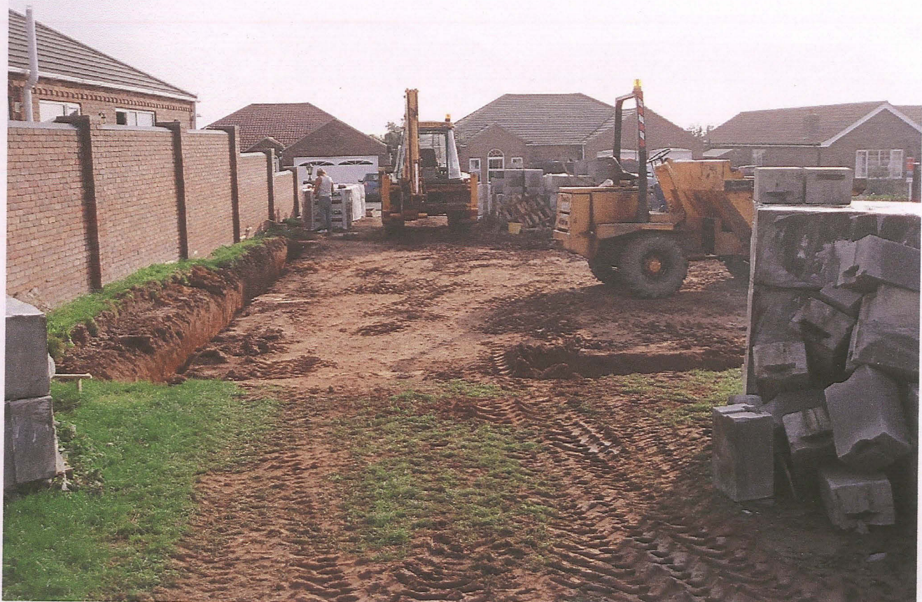
Pl. 2 Looking east across the site during groundworks
