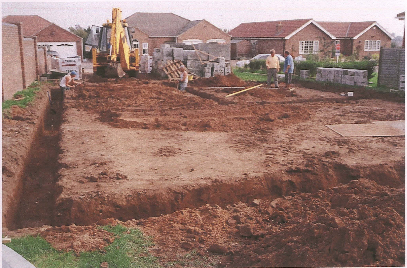
Pl. 4 Looking east at the completed footings
