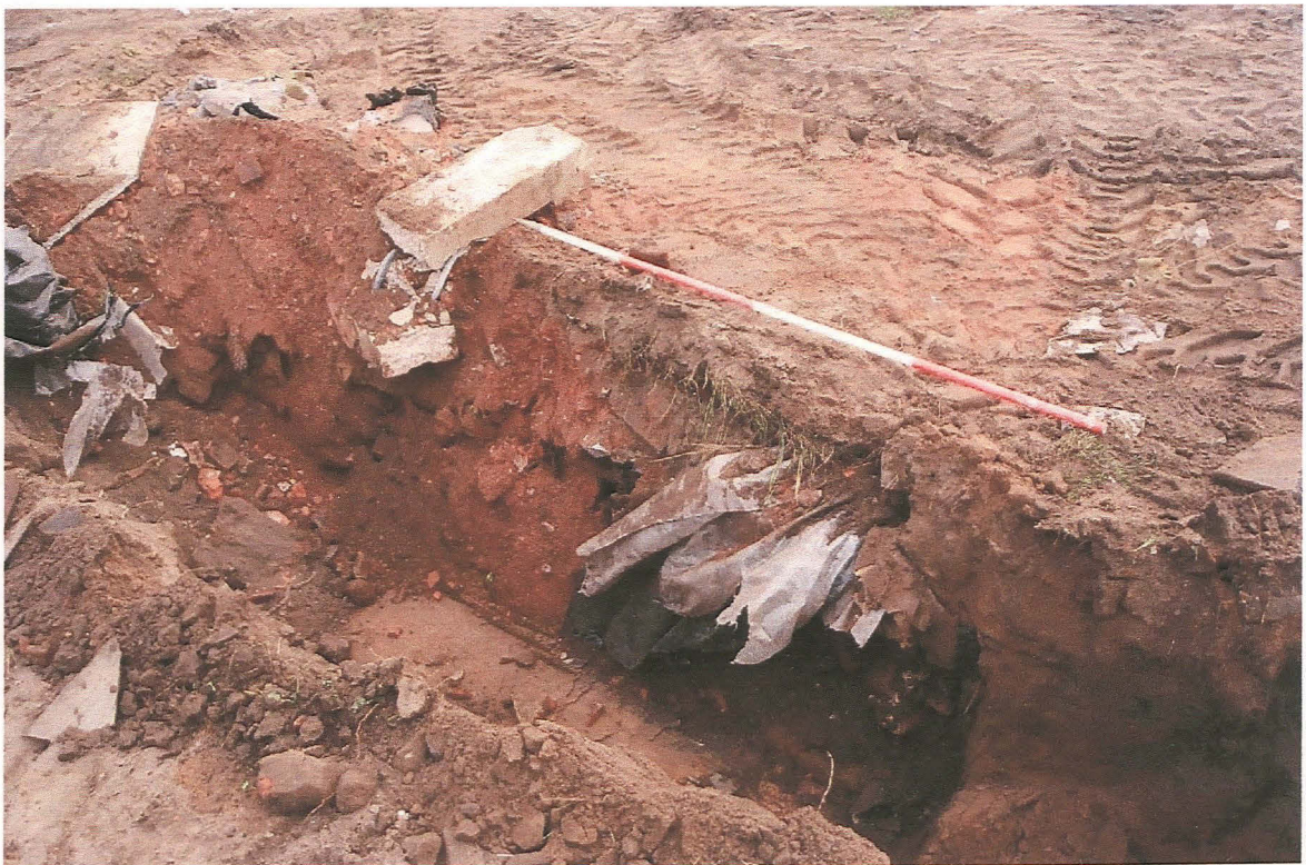
Pl. 6 Modern in-fill/pond 103, looking north-east.
