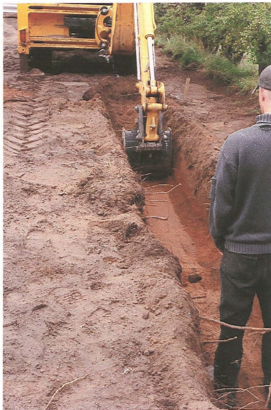
Pl. 4 Excavation of the southern external wall foundation, looking east.
