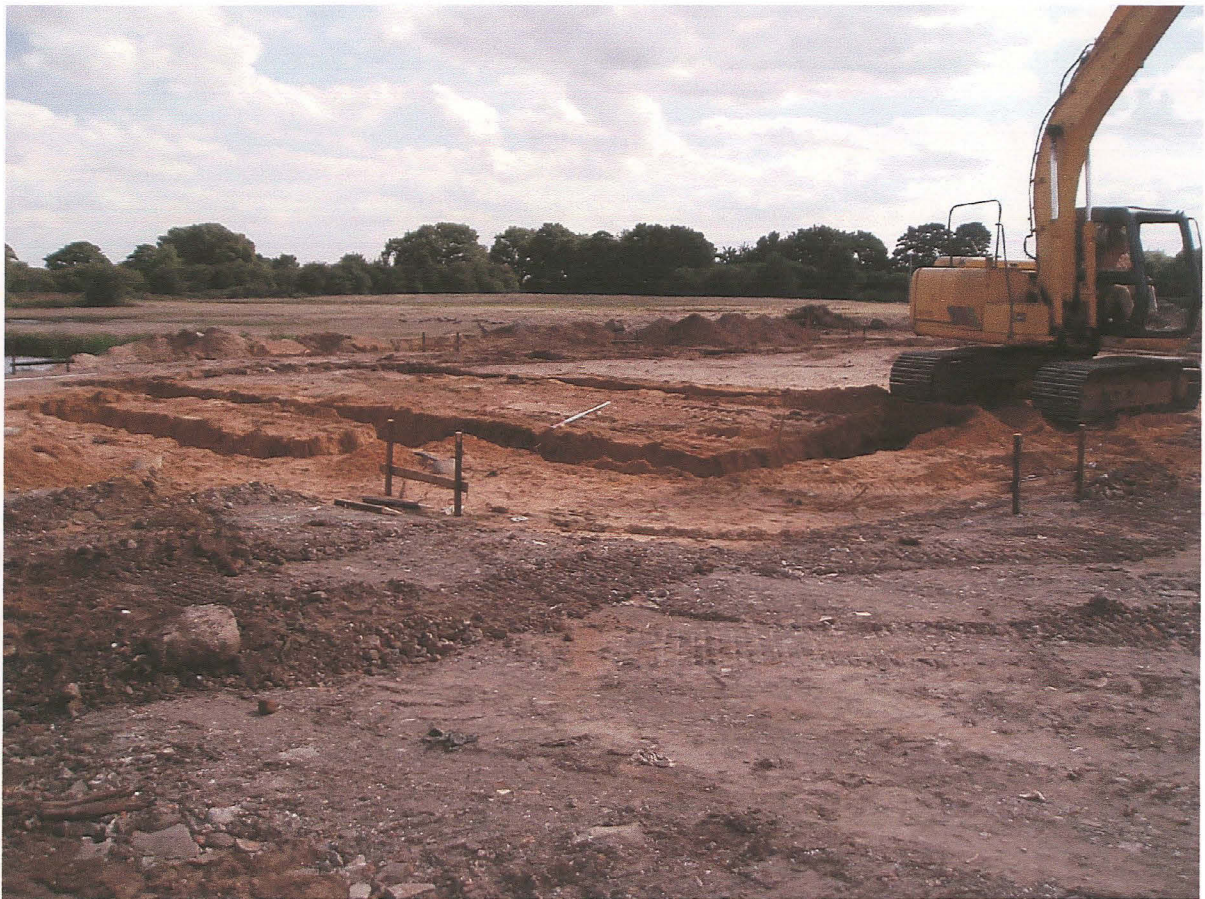
PI. 9 Machining of the house foundation trenches.
