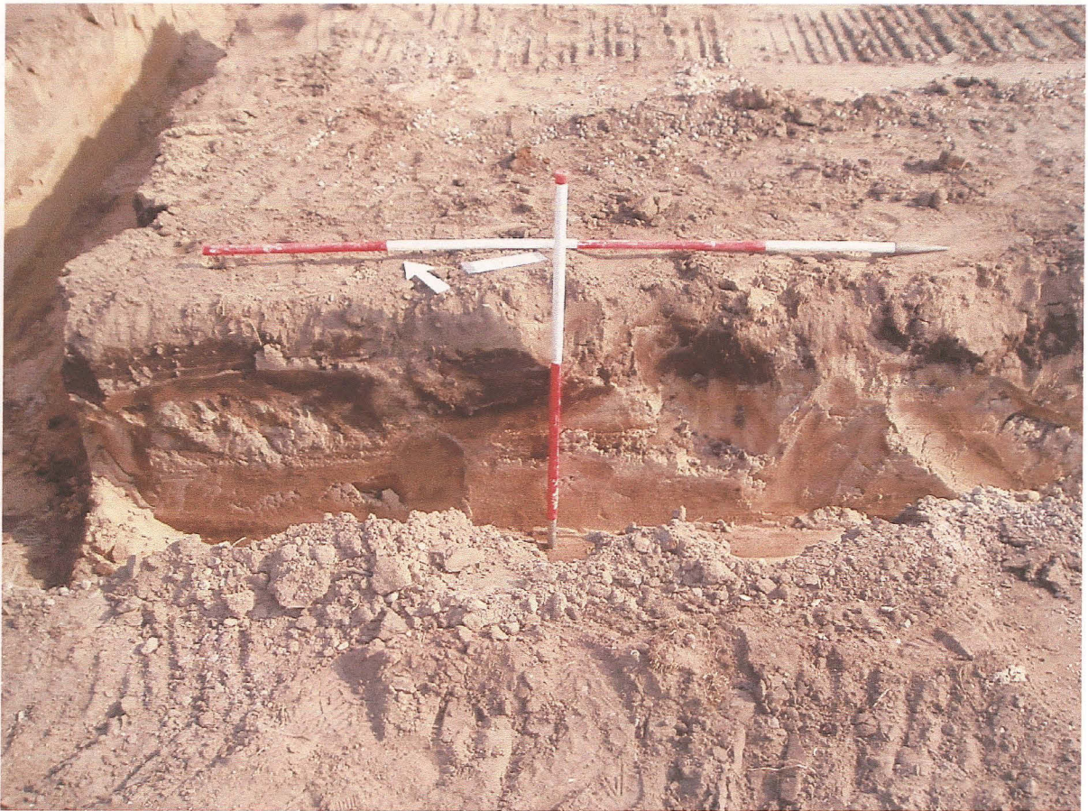
PI. 11 The north west corner of the building plot with a small amount of subsoil remaining after the stripping process.
