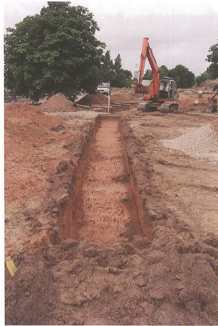
PI. 4 A section of the drains excavation trench between points A and B (see Fig. 2).
