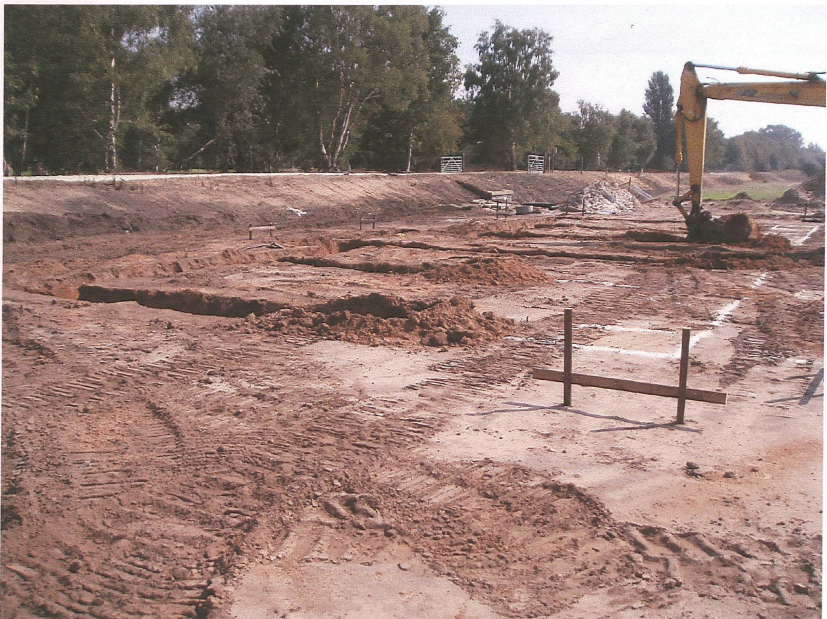
PI. 12 The foundation trenches of the garage being machined.
