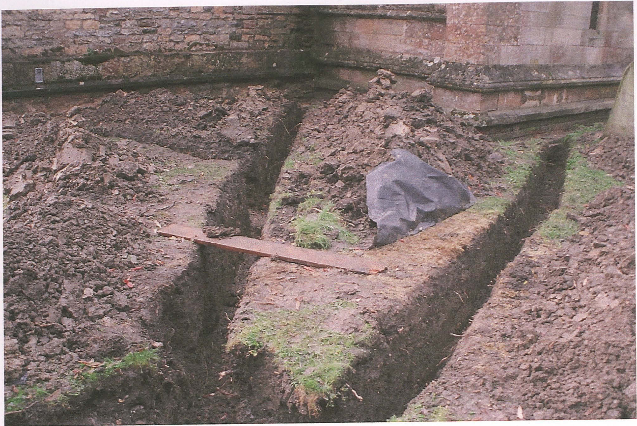
Pl. 3 Drainage trenches on the northern side of the church
