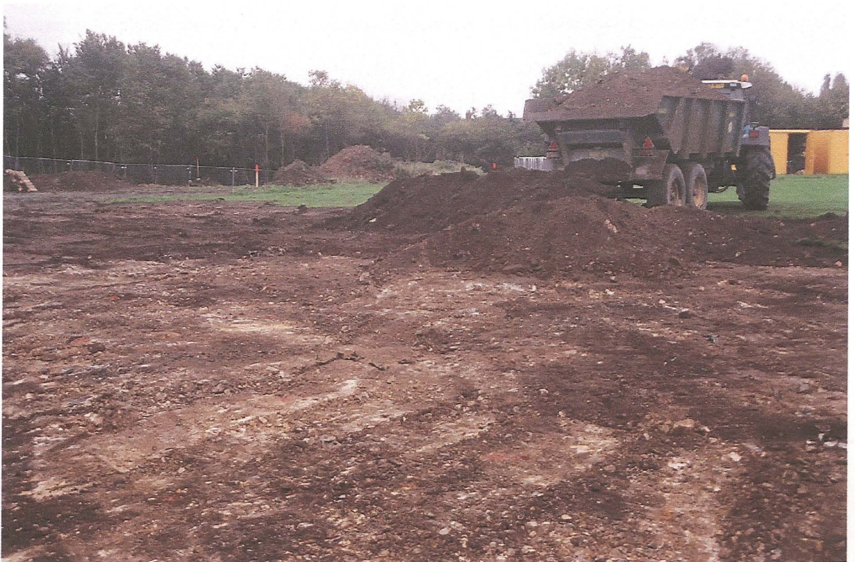
Pl. 4 West end of the site after stripping, looking south-west.
