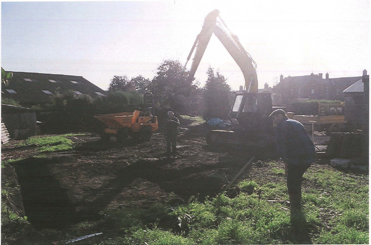
Pl. 1 The site, looking south-east across bungalow plot, with excavation in progress.
