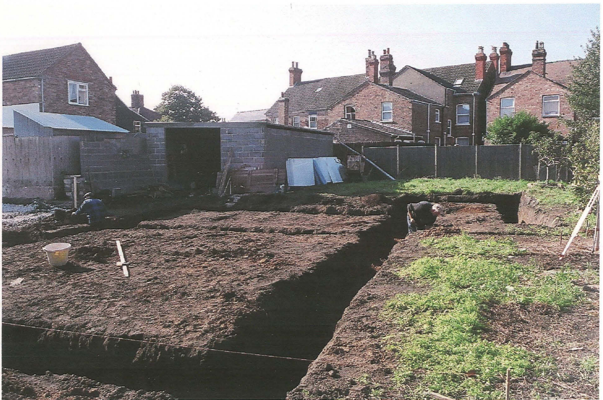
Pl. 5 Excavated bungalow plot, looking west.
