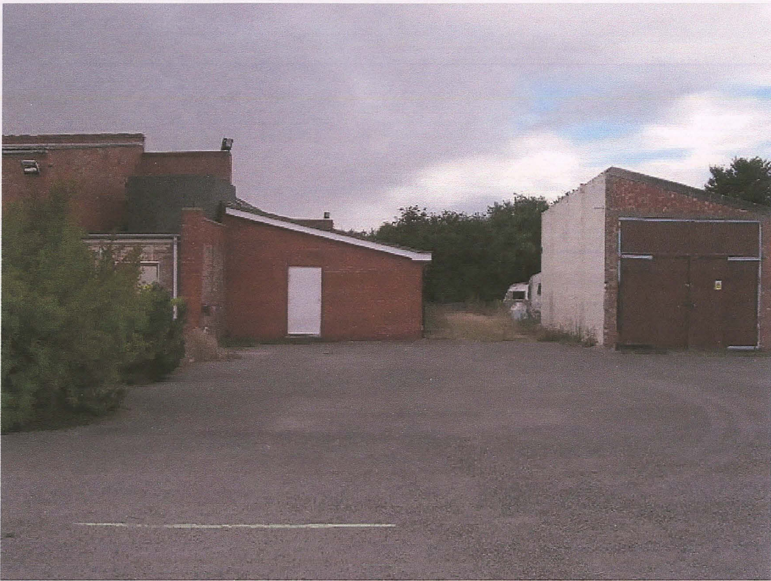
Pl. 5 Buildings at the rear of the former garage premises (looking west).
