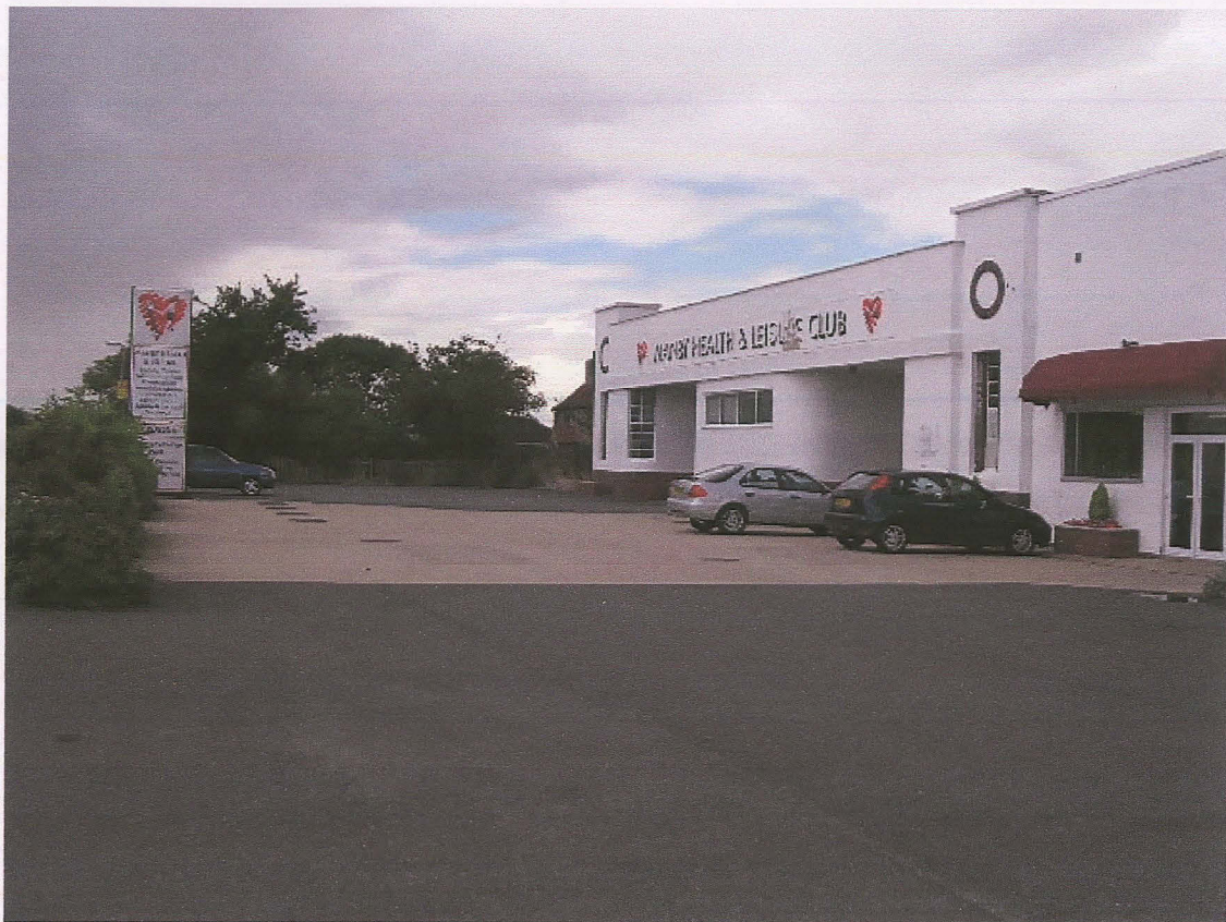
PI. 1 The former garage forecourt, showing the converted garage, the positions of underground fuel tanks, and the sites of removed pump islands (looking west).
