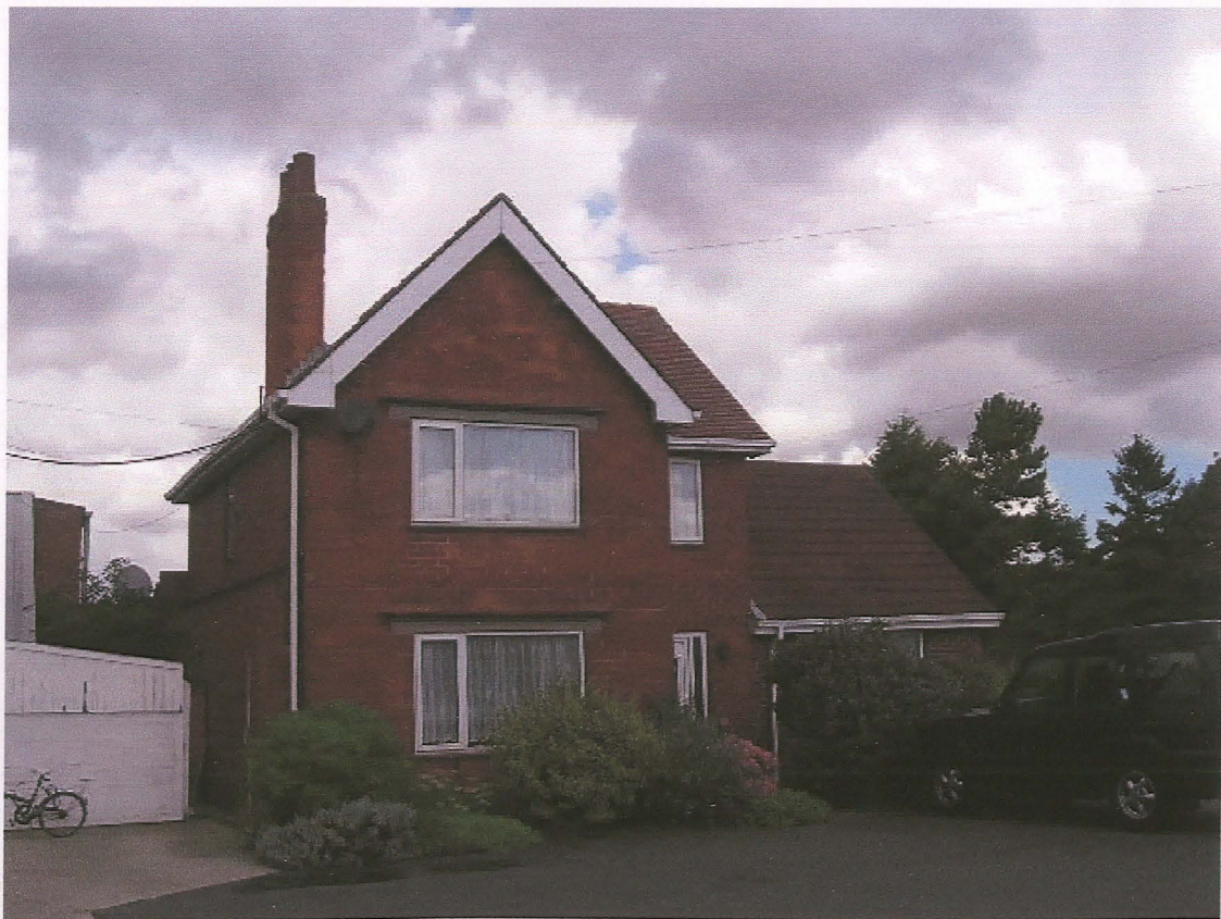
PI. 2 Front elevation of the garage house (looking north).
