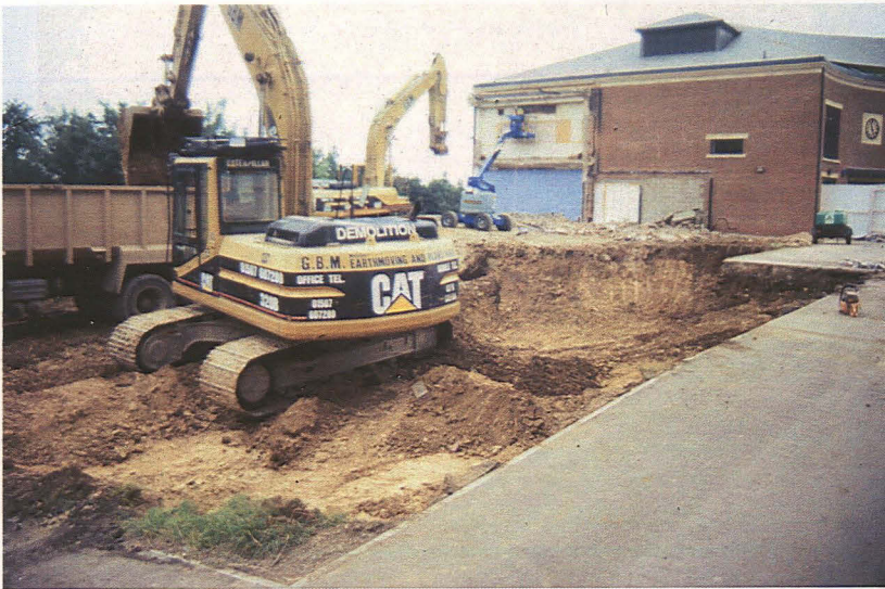
Plate 1 - View showing the ground reduction in progress, looking southwest
