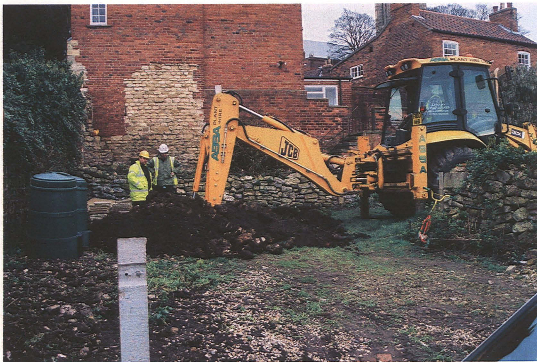
Plate 2 North facing view, showing excavation of Trench 1
