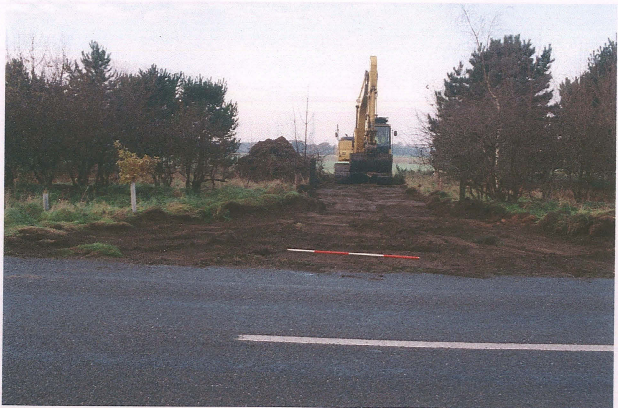
Pl. 2 General view of the access road after stripping, looking west.
