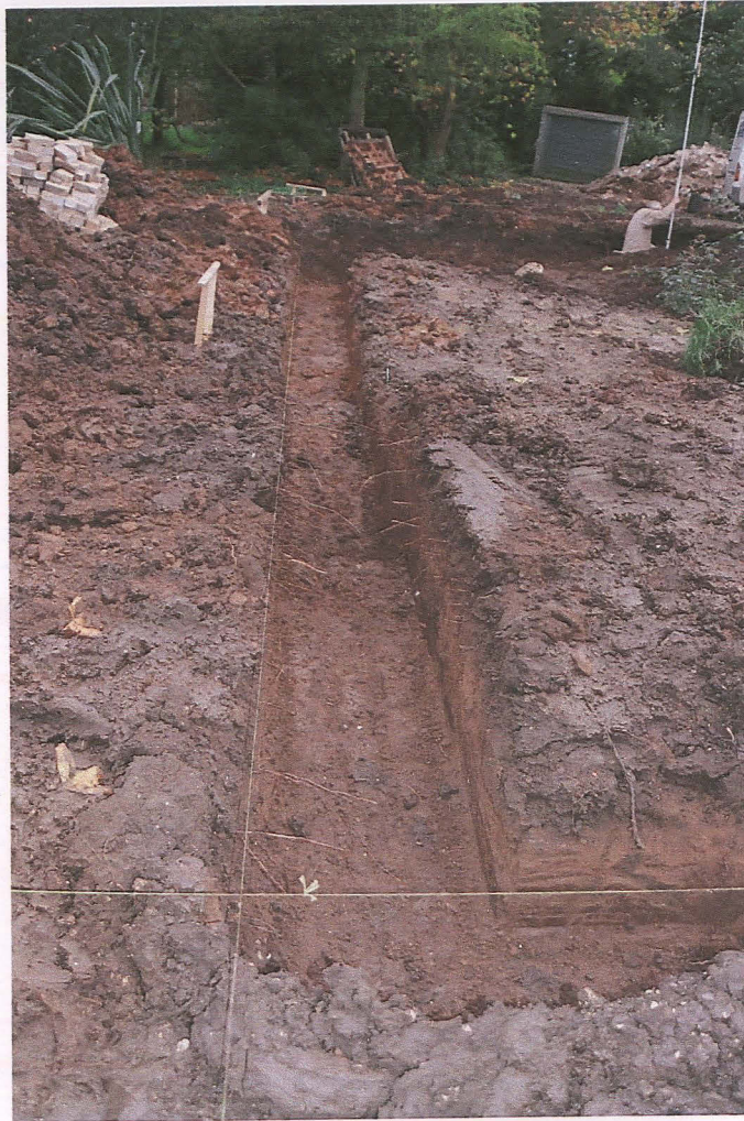
Pl. 7 View of northeast trench of extension, looking southeast.
