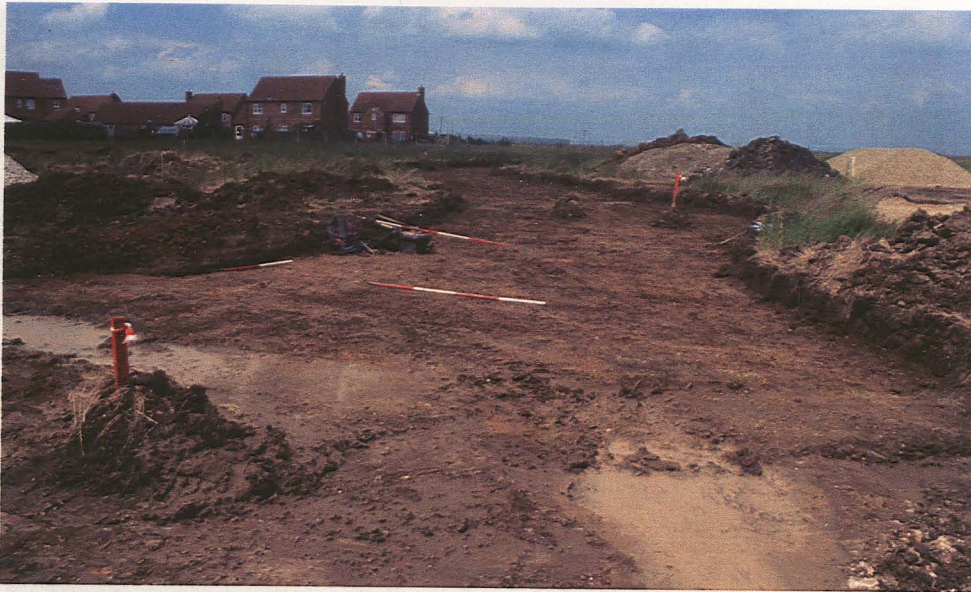
Plate 1: General shot of stripped Road 4 looking north
