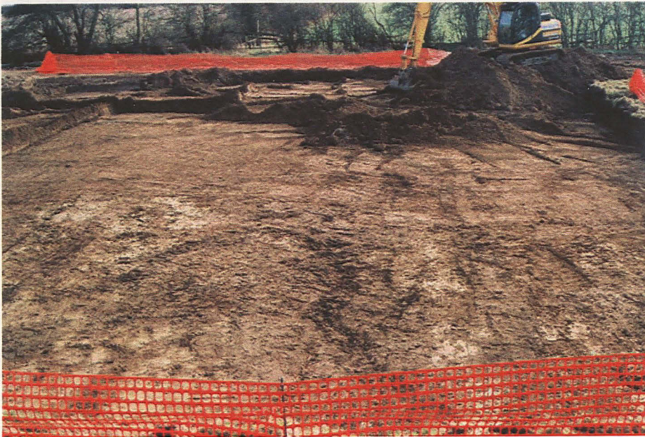
Plate 2 Site during stripping facing north
