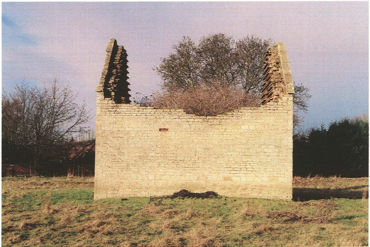
Plate 10. SE side of Dovecote
