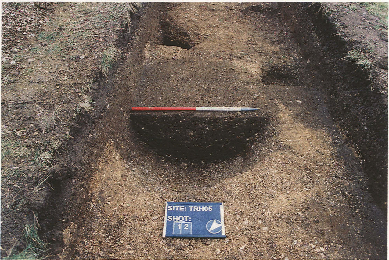
Plate 5. Trench 3, Section 14 through Pit [020] Looking SE
