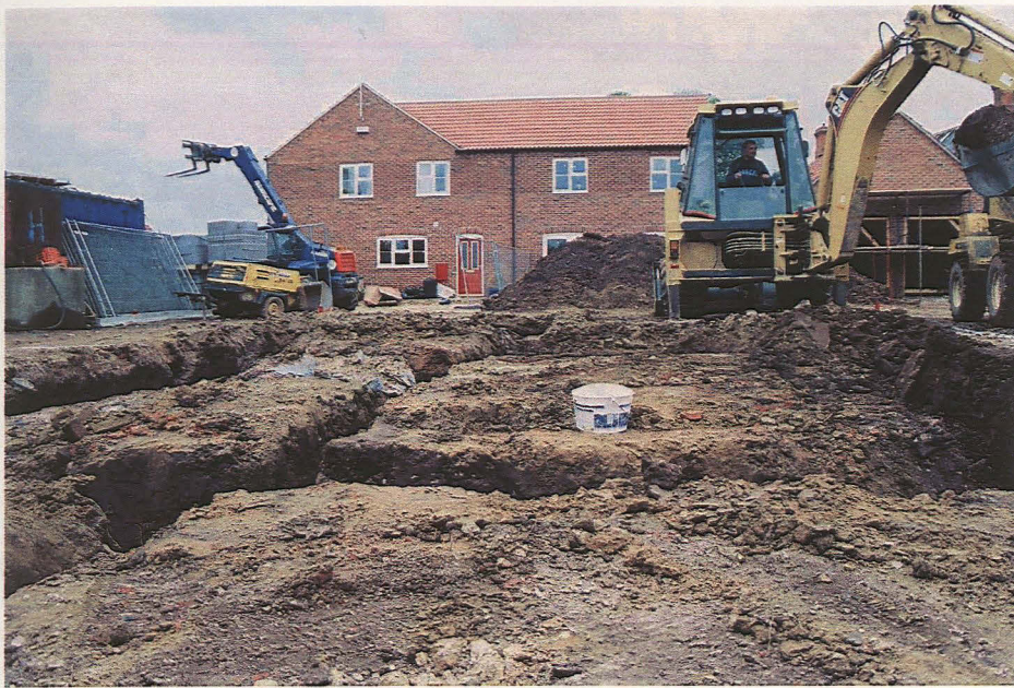
Plate 1: General view showing foundation trenches, looking west
