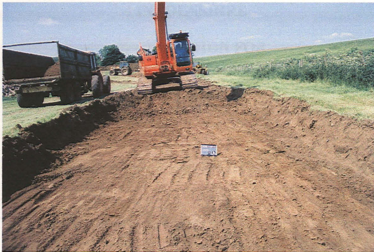
Plate 2 North facing view of Area 2
