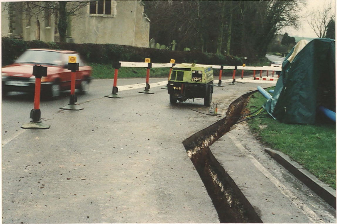
Pl. 3 Chalk rubble above sandy clay to the east of Holy Trinity Church, looking NW
