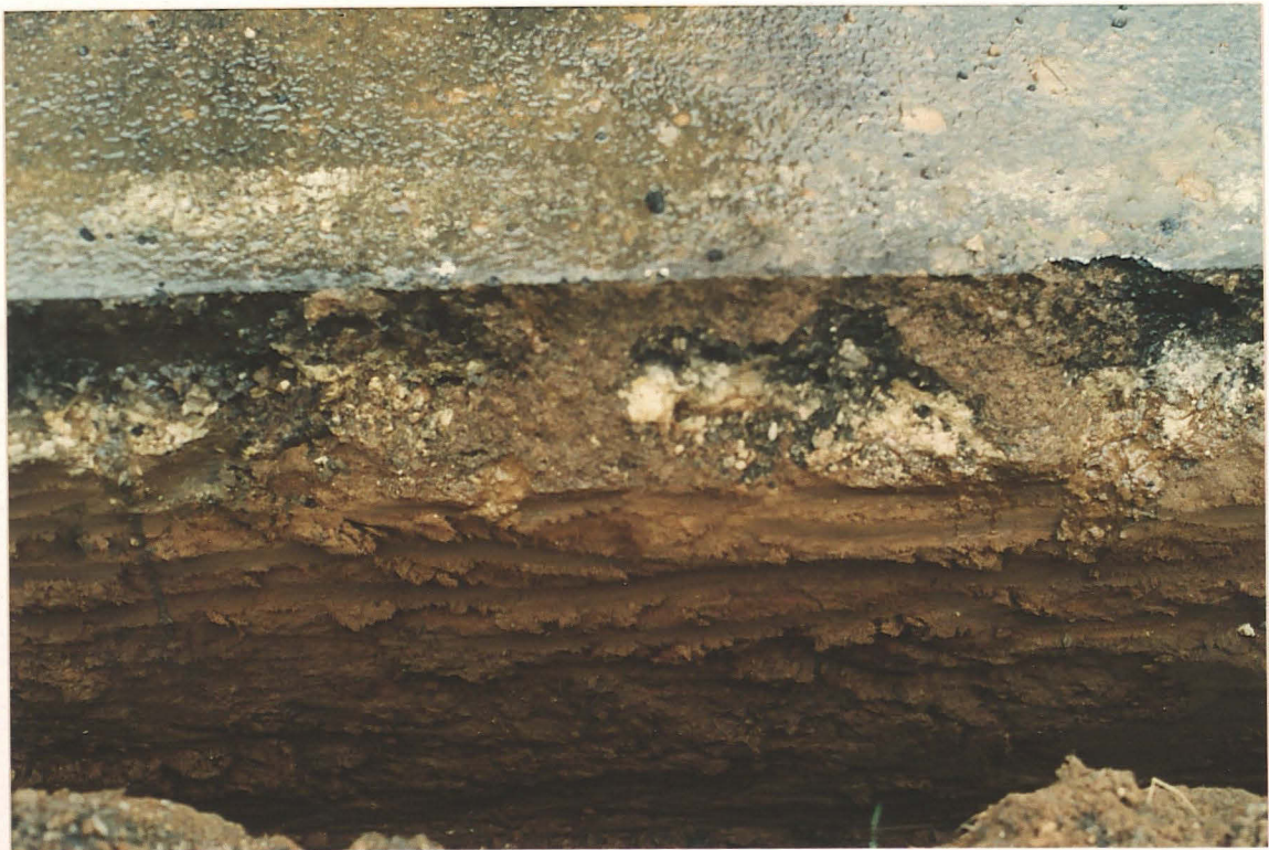
Pl. 4 Trench face close to Bilsby Church showing tarmac and chalk rubble above sandy clay subsoil
