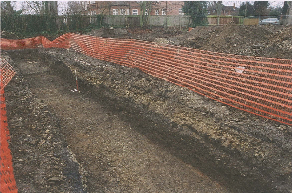
P. 7 Trench 3, north section, looking northwest.
