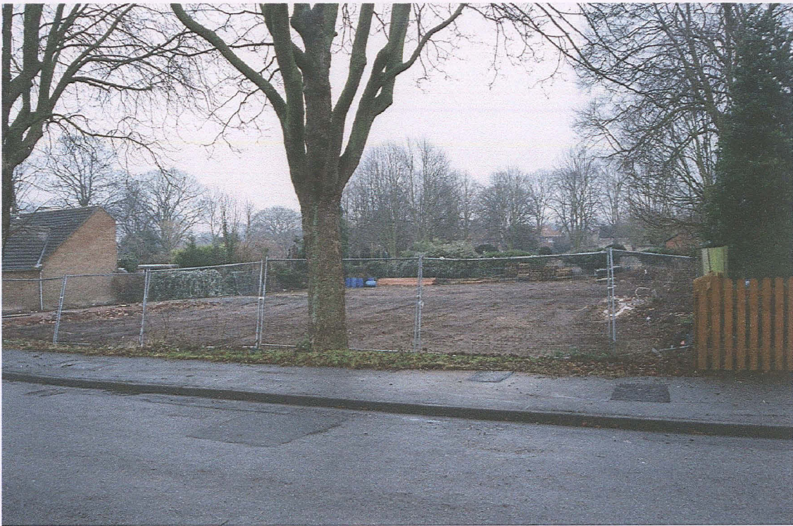
Pl. 1 View of development area looking southeast.
