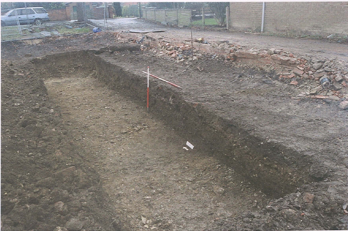
Pl. 2 View of Trench 1, looking north.
