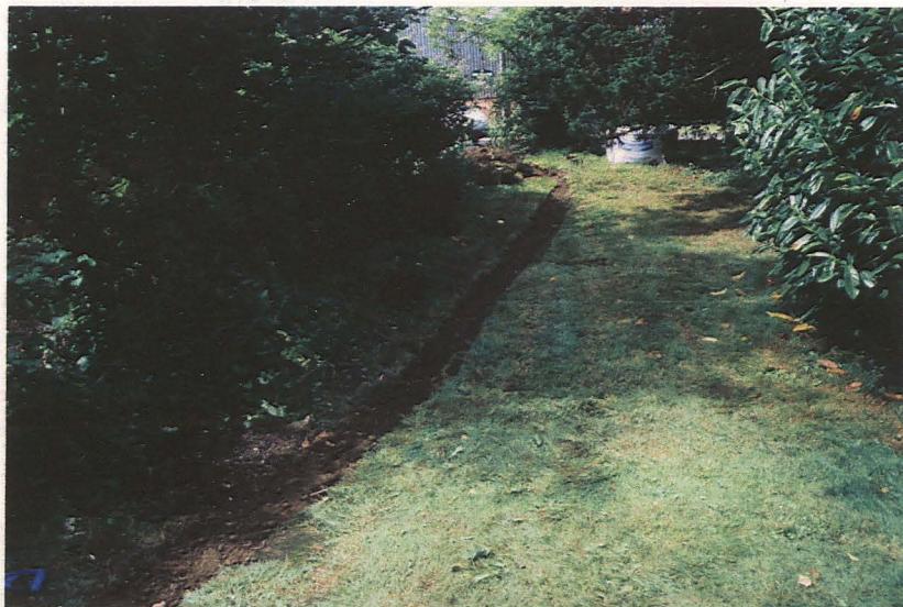
Plate 3 - View showing the backfilled trench, looking north
