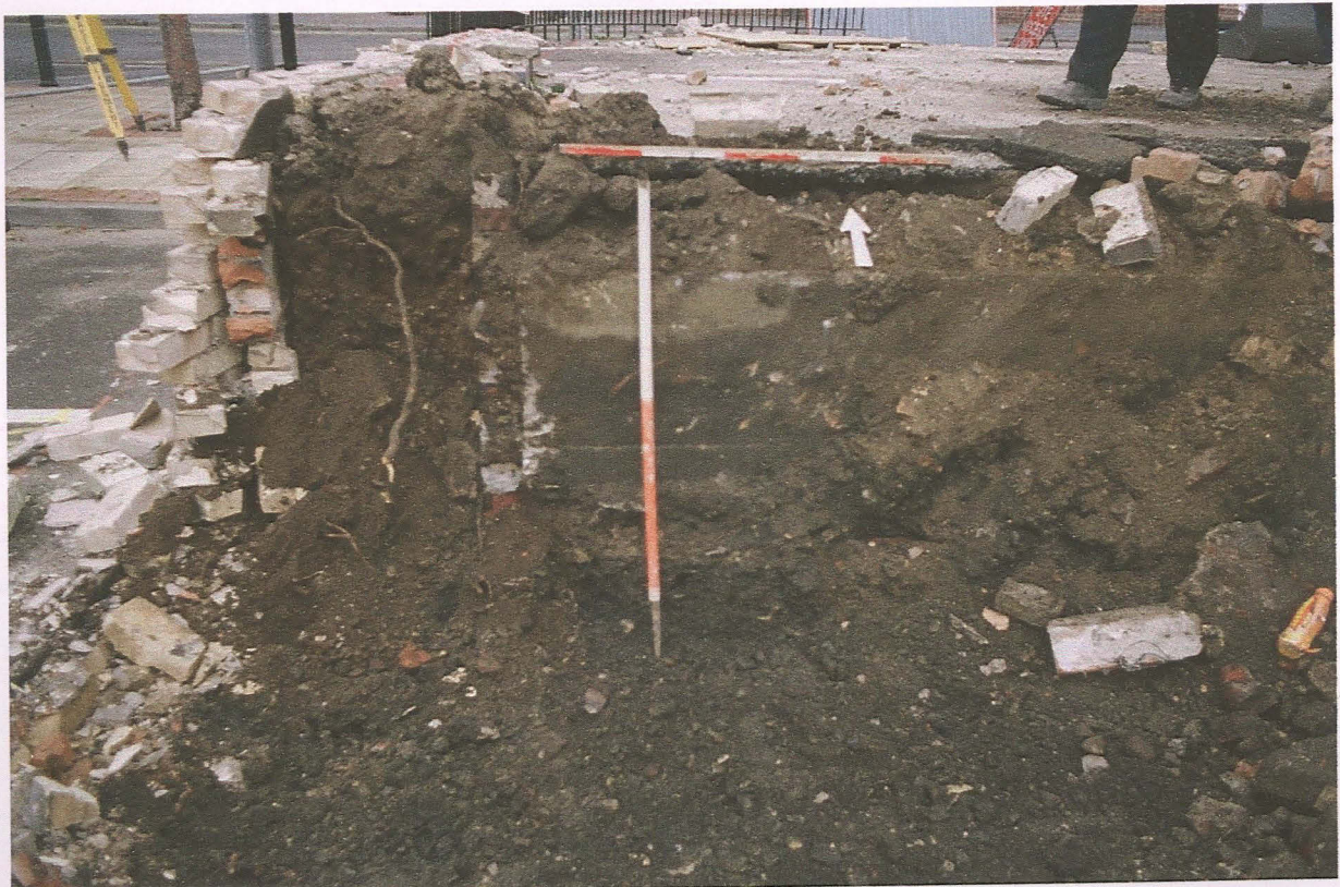
Pl. 2 Stripping of the proposed building area to a depth of c.17.00m O.D. exposed only modern deposits. Scales 1m.
