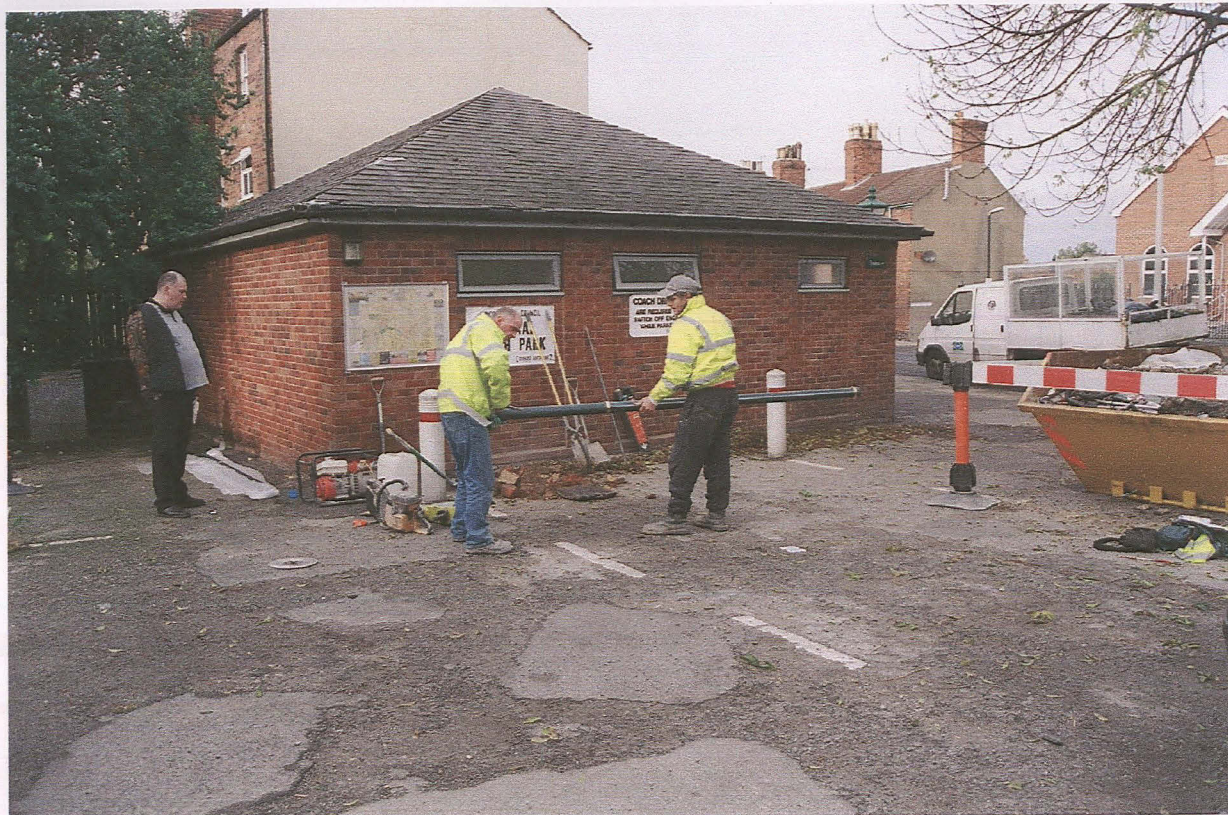
Pl. 1 Sign 6 during excavations, looking west towards Westgate public convenience.
