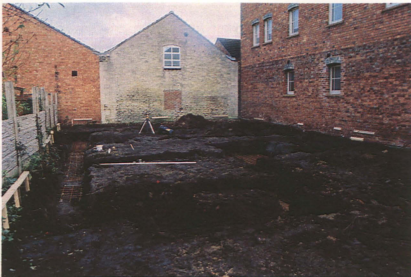
Plate 1 - View showing the development area, looking northeast
