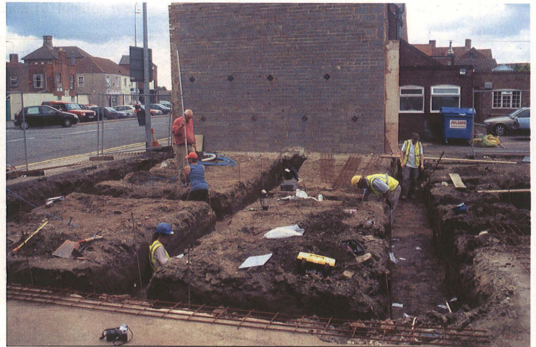
Plate 2: Plot 9 and 10 footings, looking northeast
