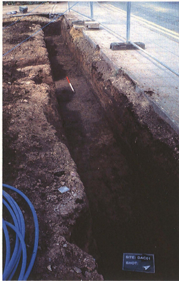
Plate 8: View of E - W northern footing, looking west
