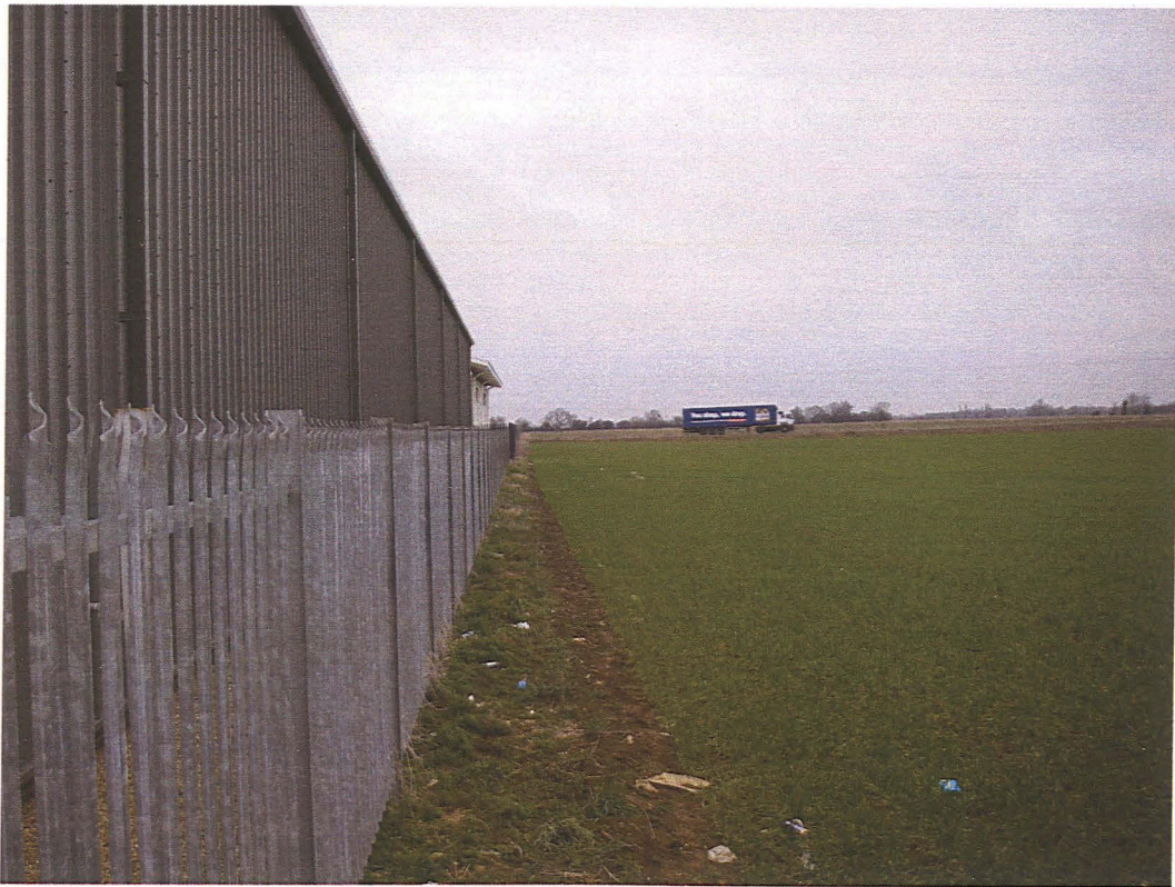
Plate 2: View of ferrous fencing and buildings facing North-West.
