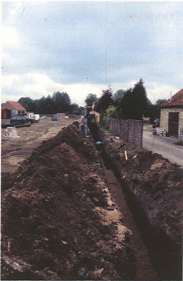
Plate 1 General view of service trench
