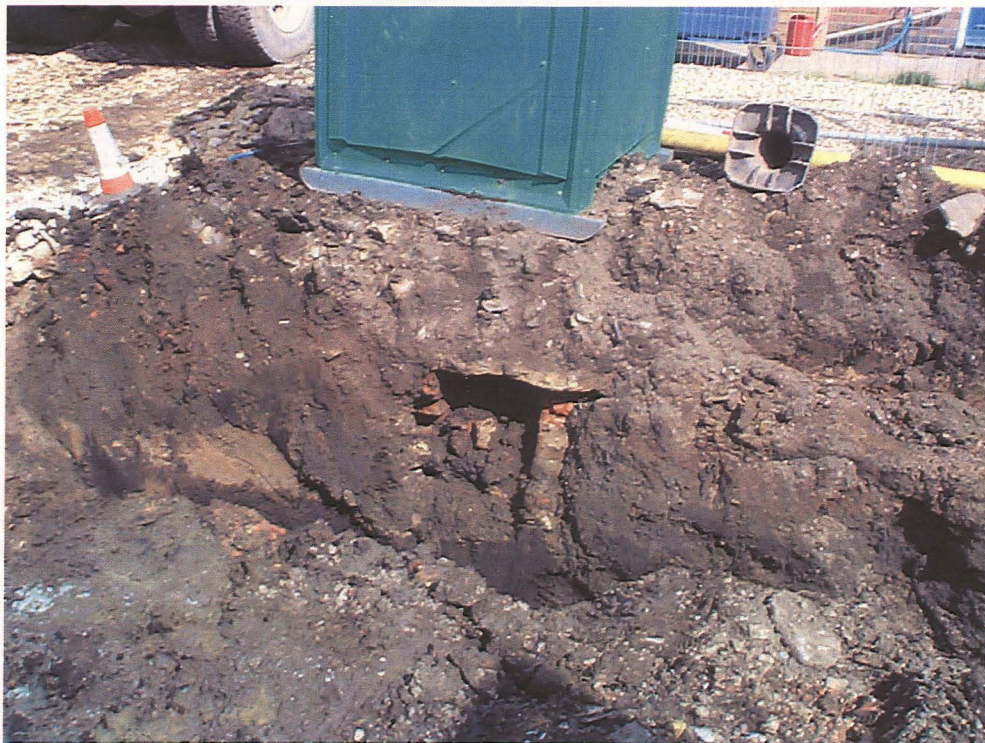
Plate 4. Stone capped culvert 015 looking east
