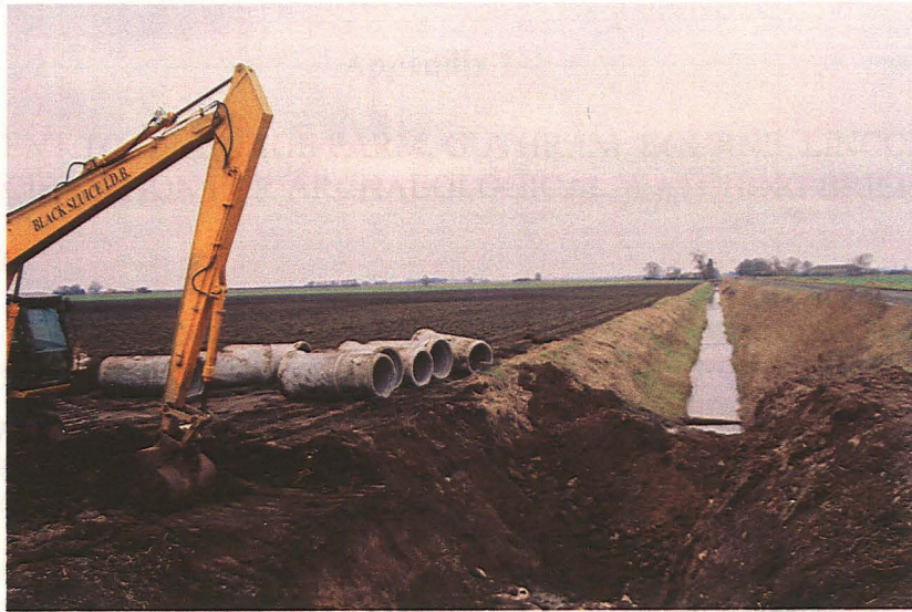
Plate 1 - View showing the drainage works in progress, looking southwest
