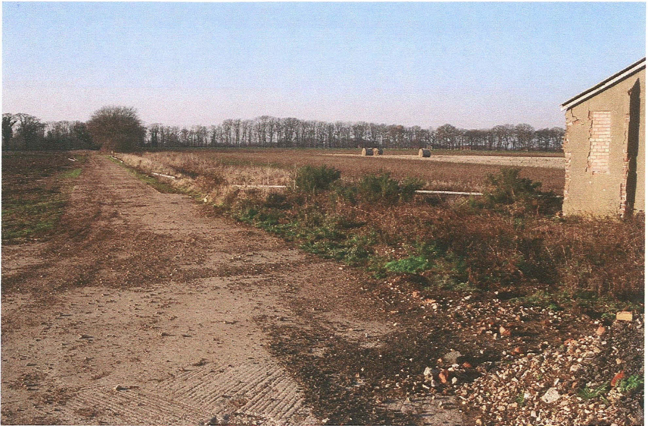
PI. 9 Concrete road, linking two demolished groups of wartime buildings, probably associated with RAF Woodhall Spa airfield (looking west towards the plantation belt).
