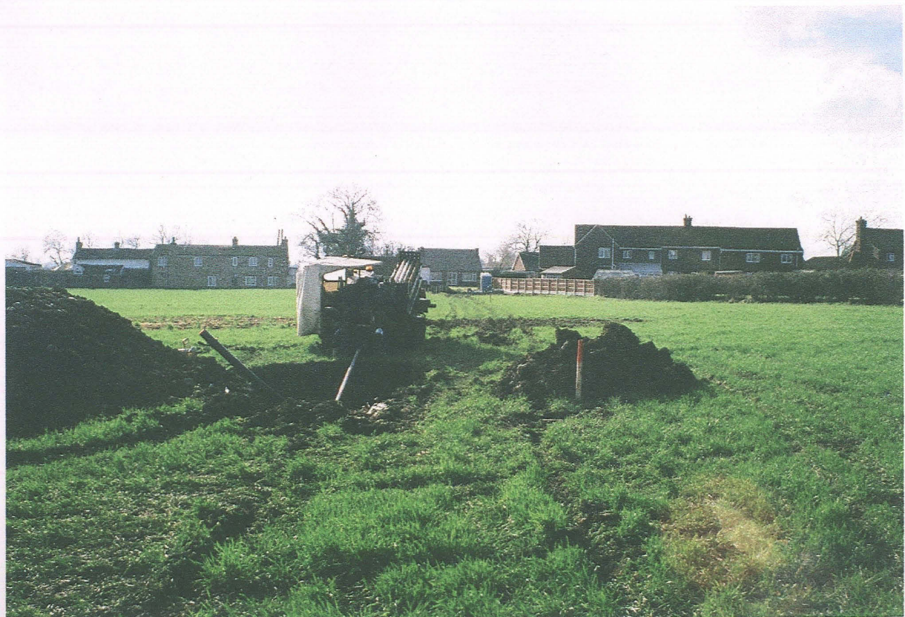
Pl. 2 Looking South at observation pit 2 during the drilling process
