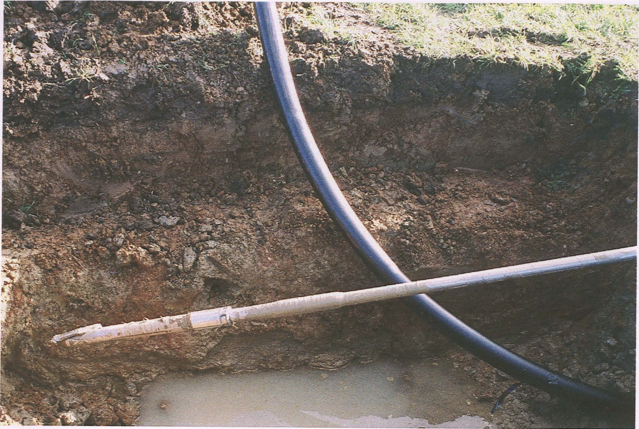
Pl. 3 Looking east at the section of observation pit 4 with the exposed drilling tip in the foreground
