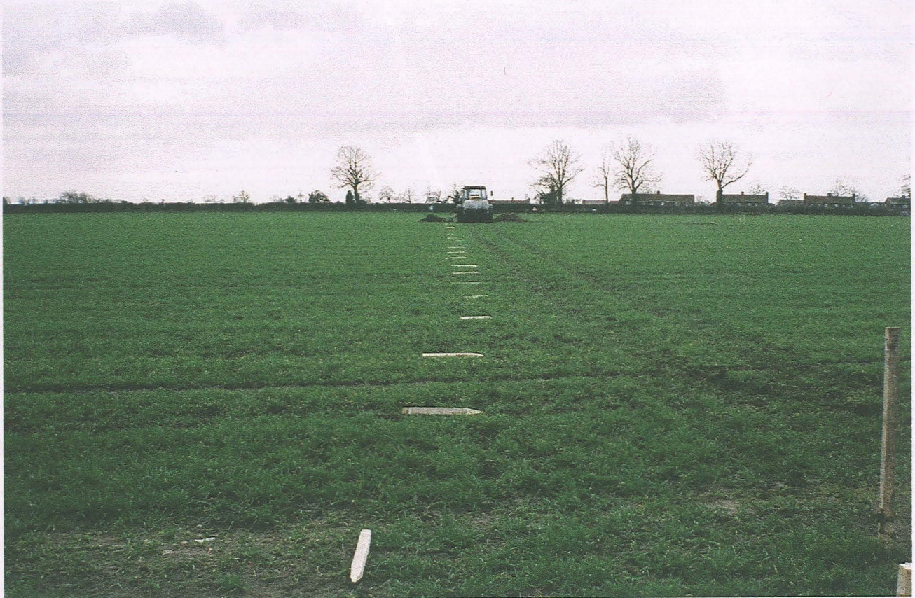
Pl. 1 Looking south along the line of the works towards Kexby
