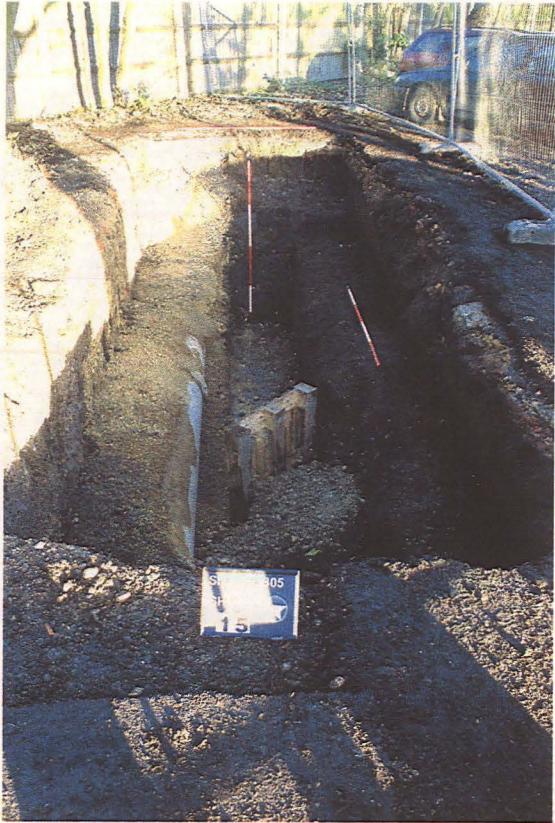
Plate 3 - Trench A after cleaning, looking northeast
