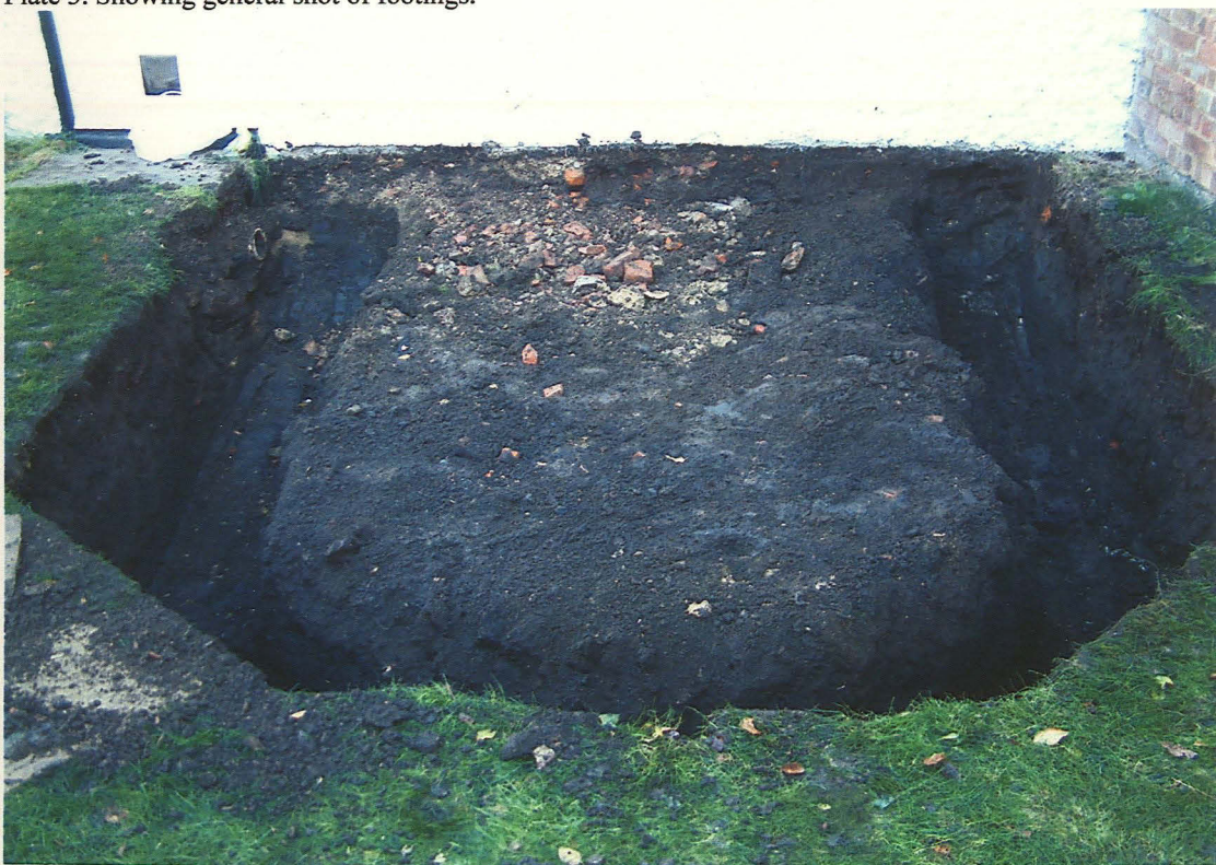
Plate 4. Showing finished footings for conservatory.
