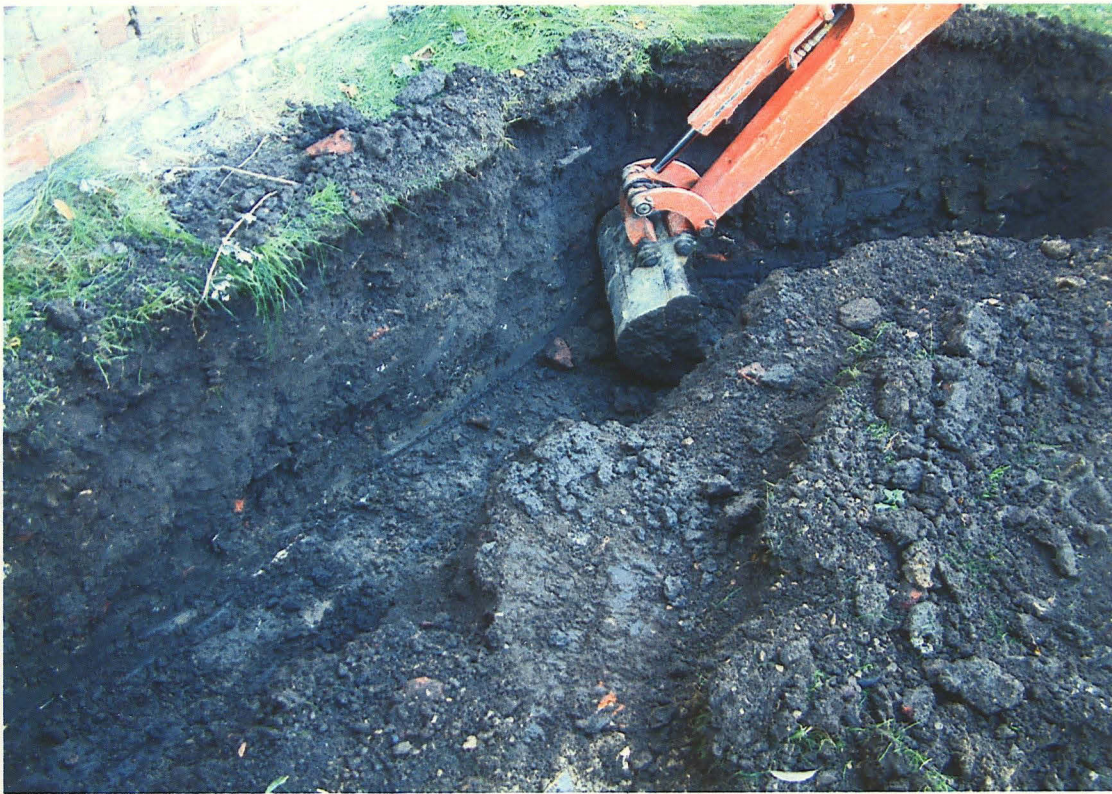
Plate 3. Showing general shot of footings.
