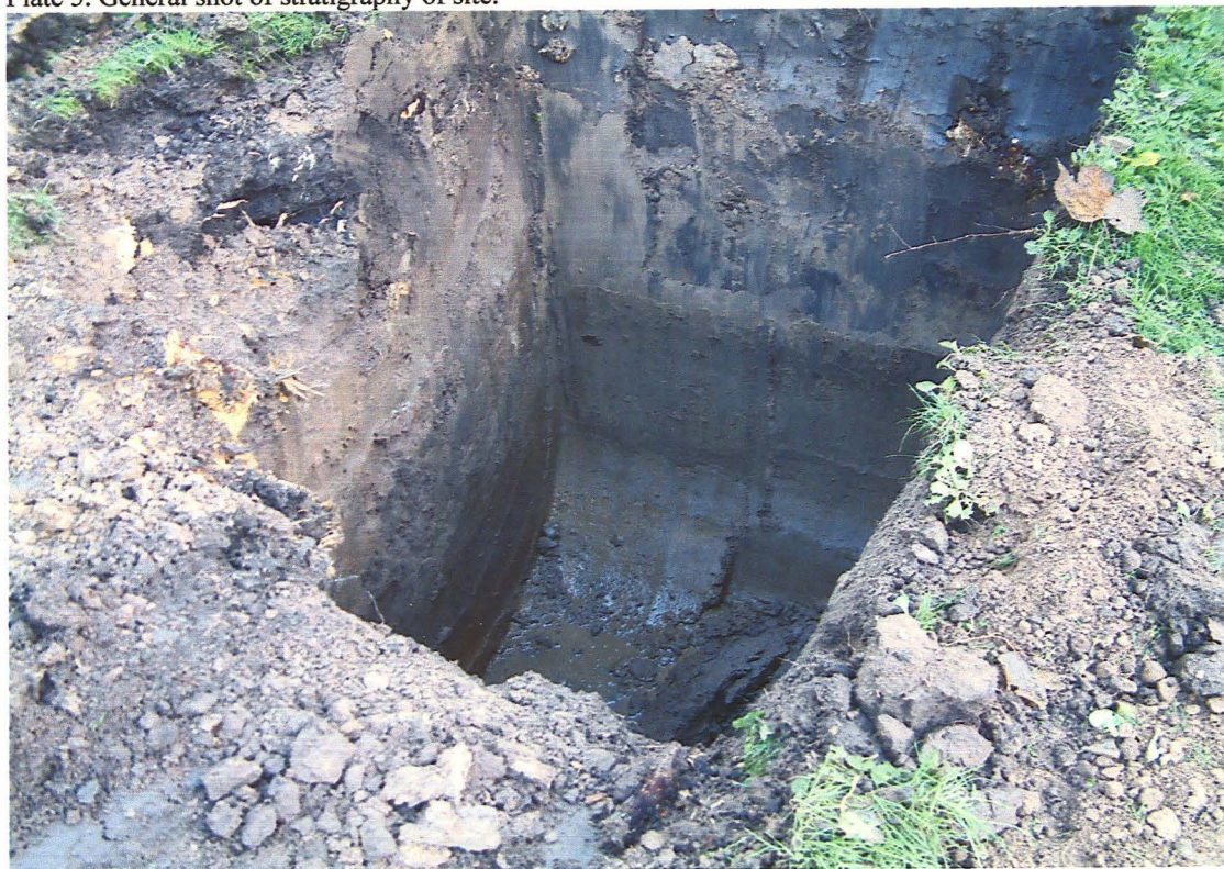
Plate 6. New soakaway for drainage in north of site.
