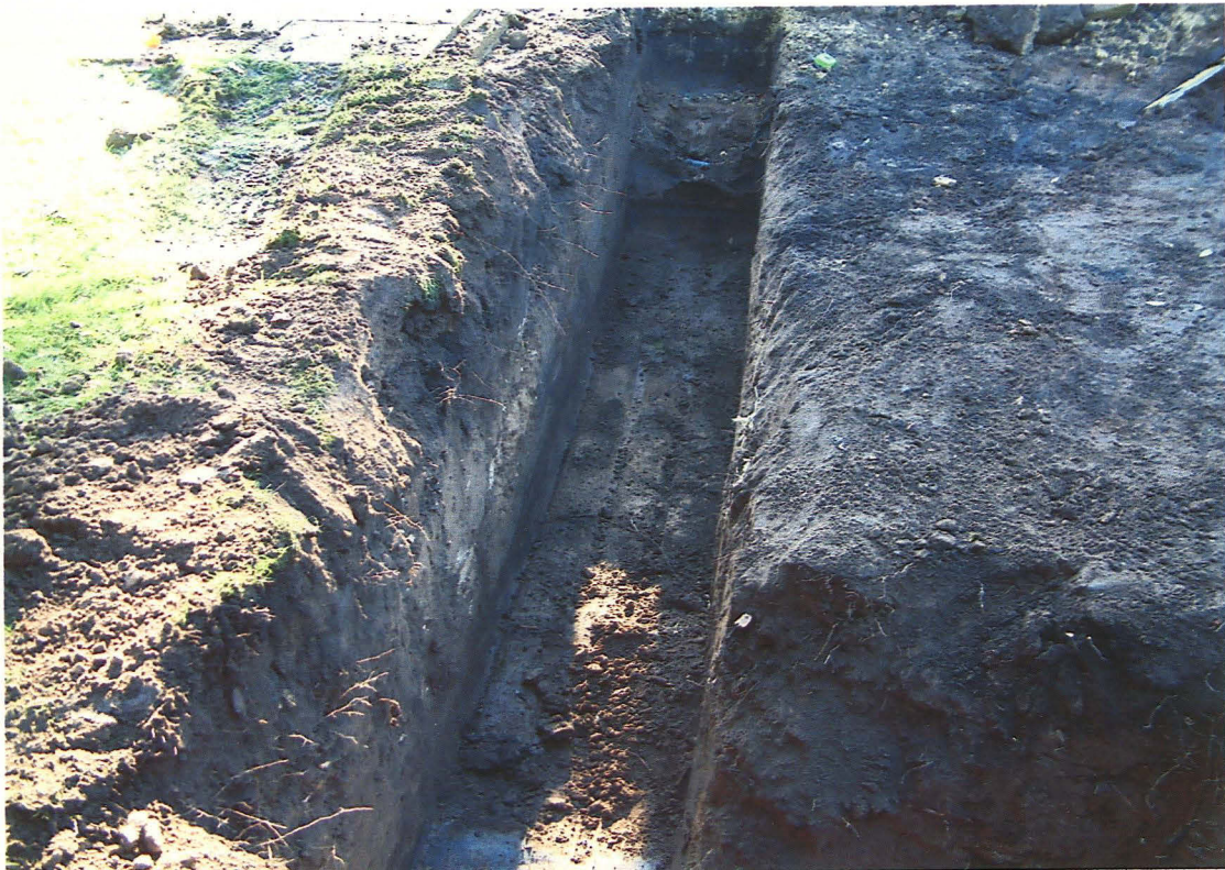
Plate 3. Showing footings through made up ground looking south.
