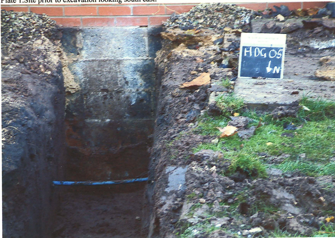
Plate 2. Showing depth of footings and water pipe.
