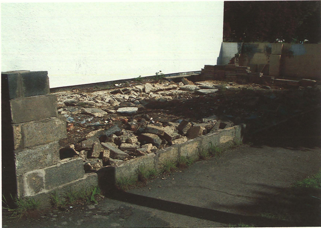
Plate 1. Site looking south east prior to clearance.
