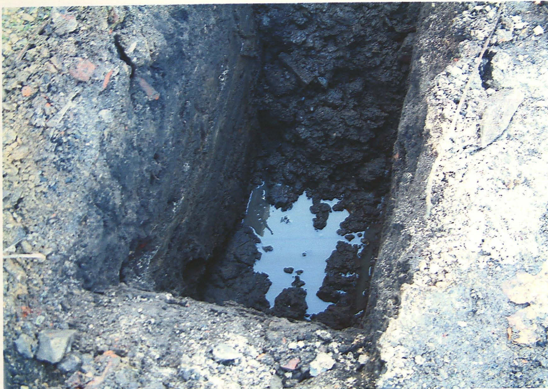
Plate 3. Initial footing in east of site showing made up ground and water table.
