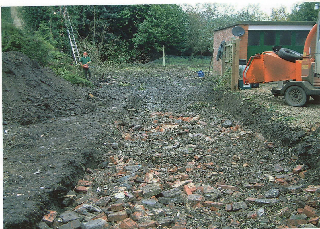
Plate 1. Site looking north showing old wall used as footings for new drive.
