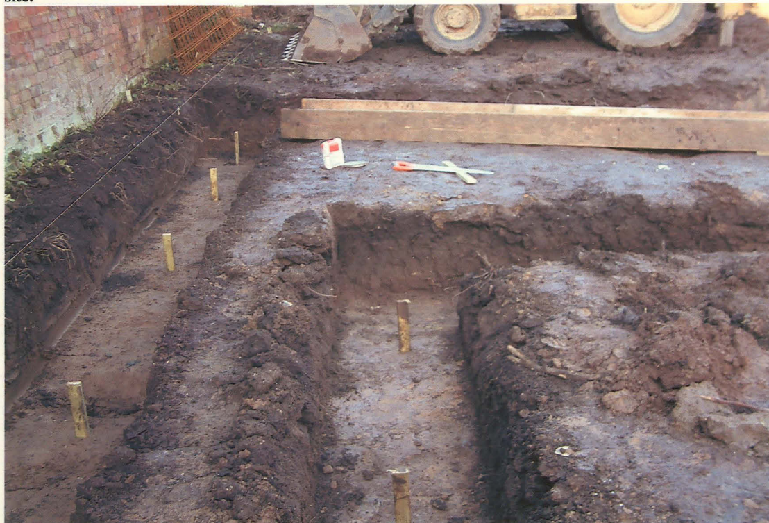
Plate 8. Showing average depth of footings.
