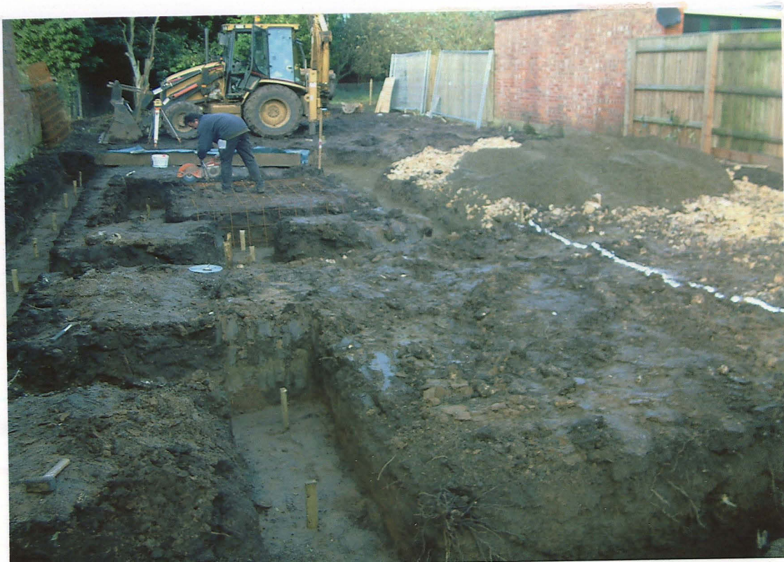
Plate 5. General shot of footings for new build.
