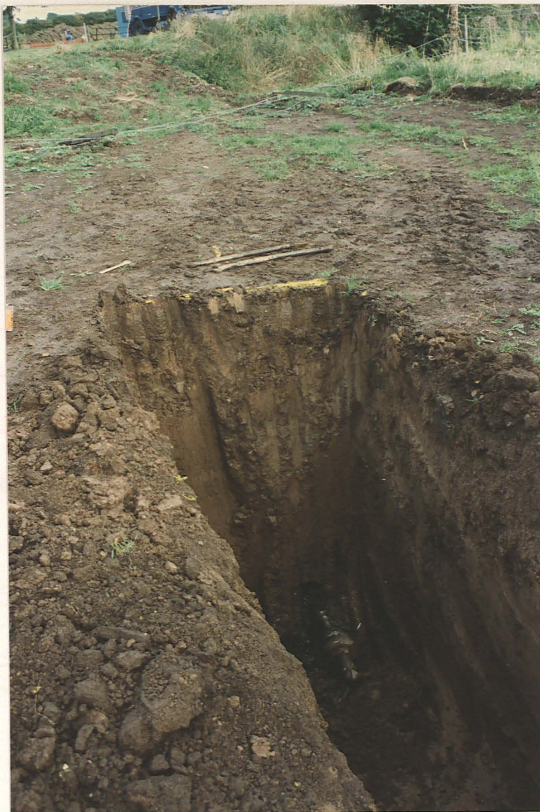
Pl. 5 Implement for moling below the A158, penetrating within the flood silt layer. Field 2, looking east to Field 3 across the raised level of the main Skegness road.
