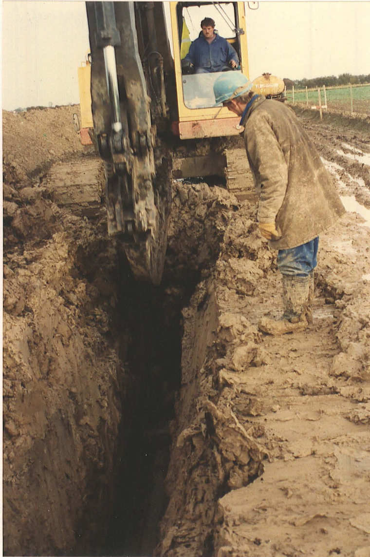
Pl. 17 Peat at the trench base, Field 23. Looking east.
