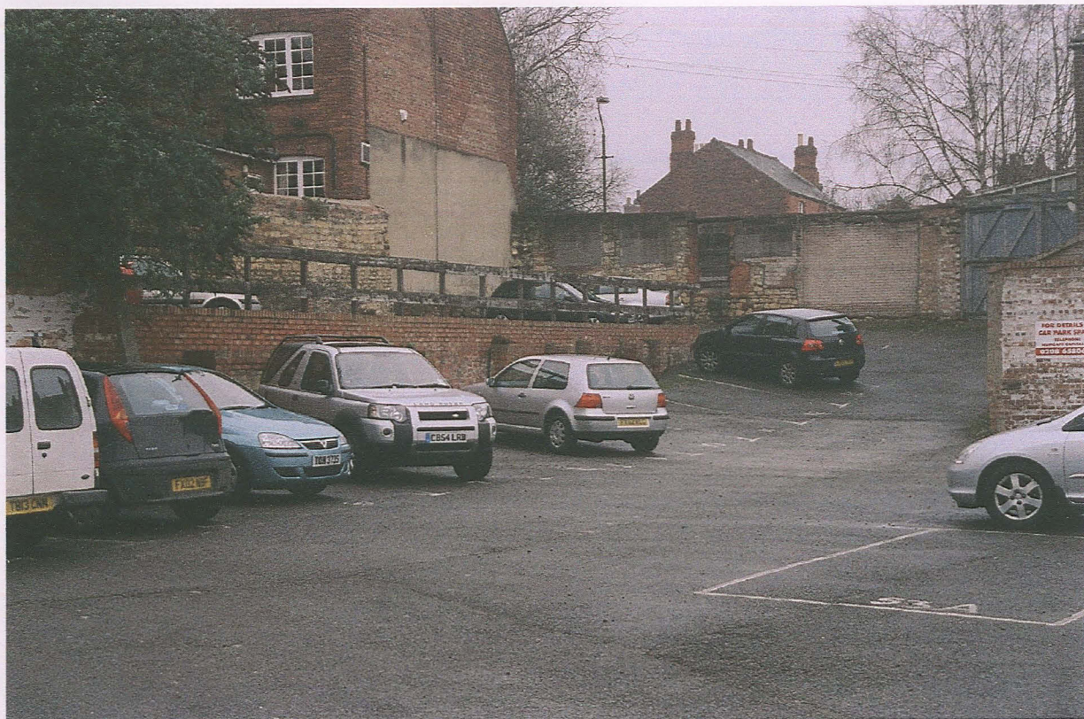
PI. 2 The car park looking northeast towards Hungate showing the current terrace walls. (06/23/28)
