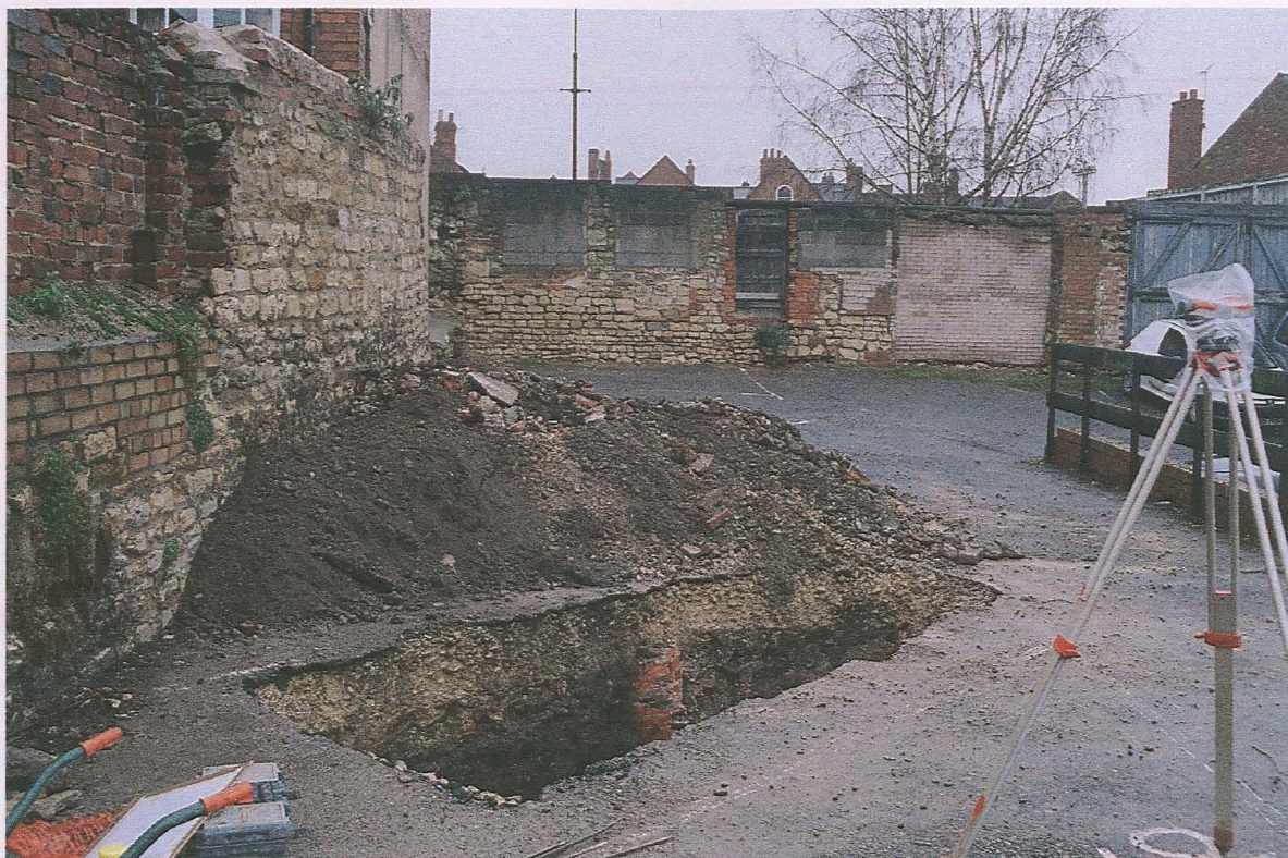
PI. 3 The evaluation trench during excavation looking east towards Hungate. (06/17/6A)
