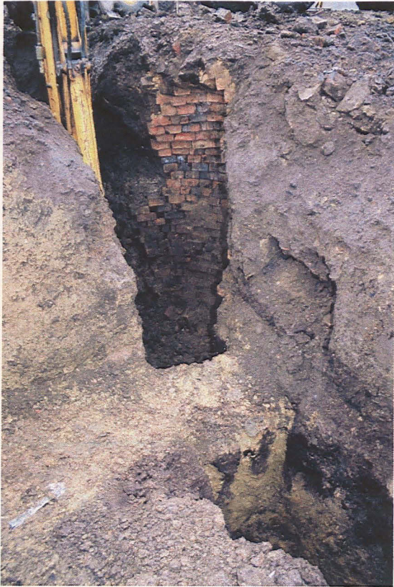
Plate 7 - Post-medieval well (179), looking northwest
