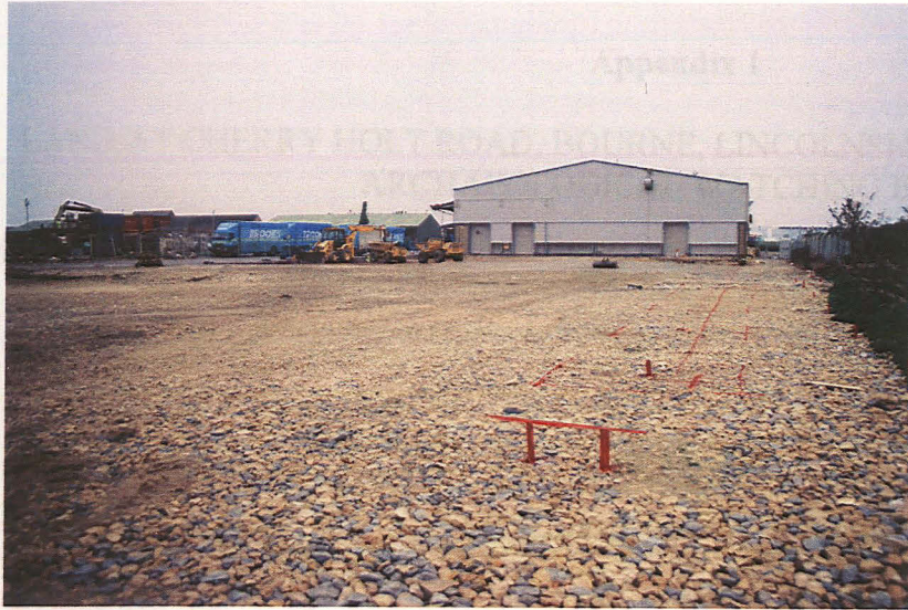
Plate 1 - General view across the site, looking north
