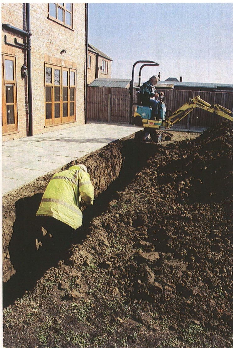
Plate 1 General Site View, looking northeast
